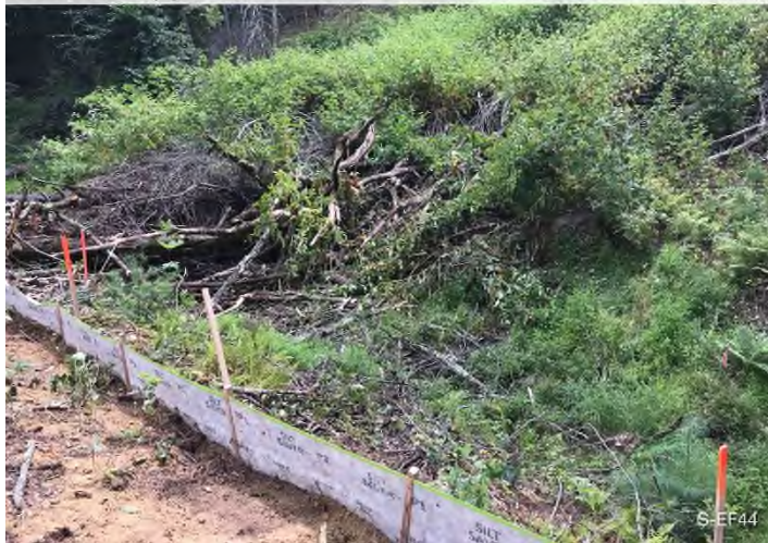
Figure 3: Stream S-EF44/Wetland W-EF44 – PPL crews installing ECDs and establishing buffer for resources.
