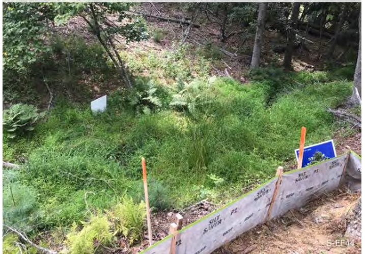
Figure 4: Stream S-EF44/Wetland W-EF44 – PPL crews installing ECDs and establishing buffer for resources.
