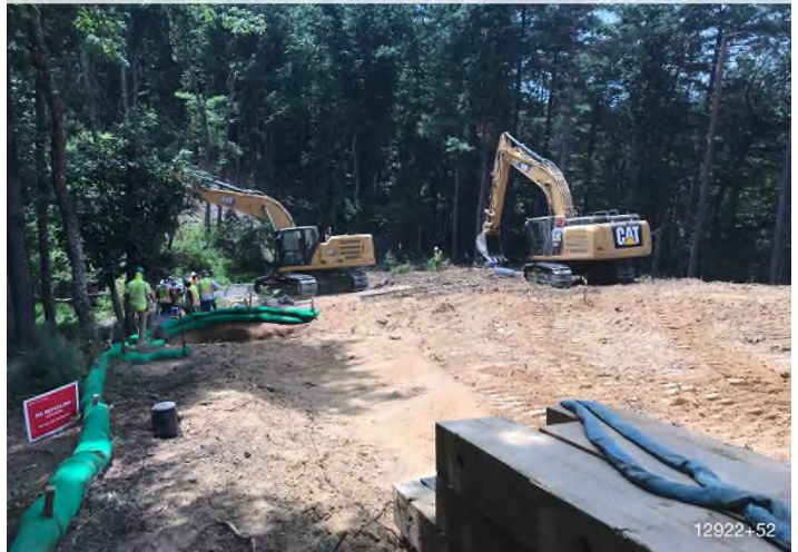
Figure 8: STA 12922+52 – Controls in place and functioning properly above stream S-EF44. PPL crews actively installing ECDs and establishing buffer area.
