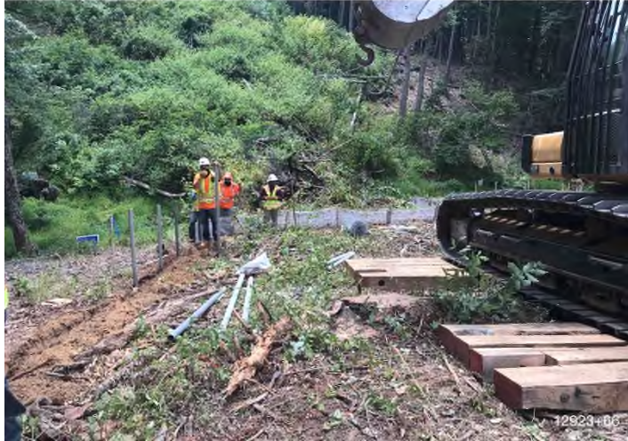
Figure 3: Stream S-EF44/Wetland W-EF44 – PPL crews installing ECDs and establishing buffer for resources.
