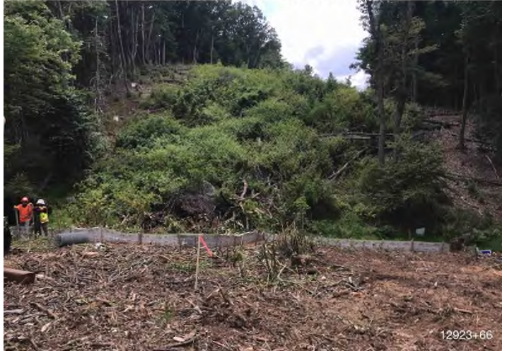
Figure 4: Stream S-EF44/Wetland W-EF44 – PPL crews installing ECDs and establishing buffer for resources.
