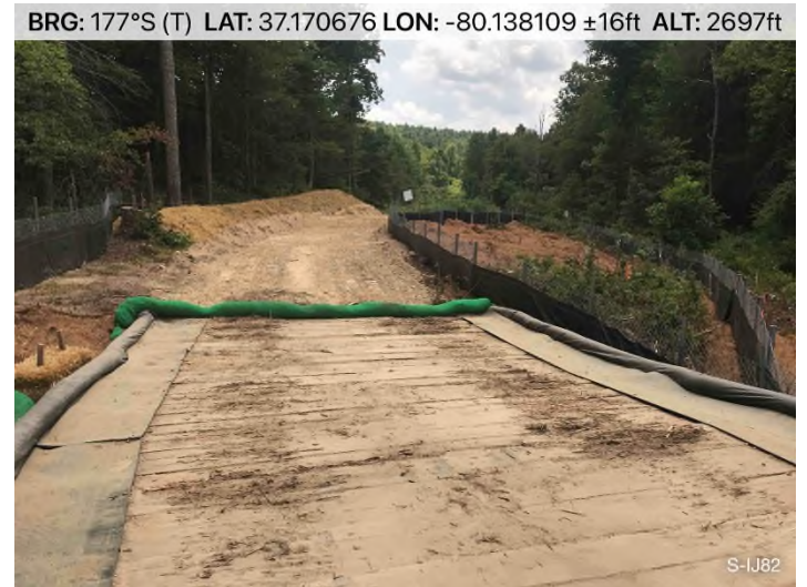
Figure 8: Stream S-IJ82 – Controls in place and functioning properly along stream S-IJ82 crossing.
