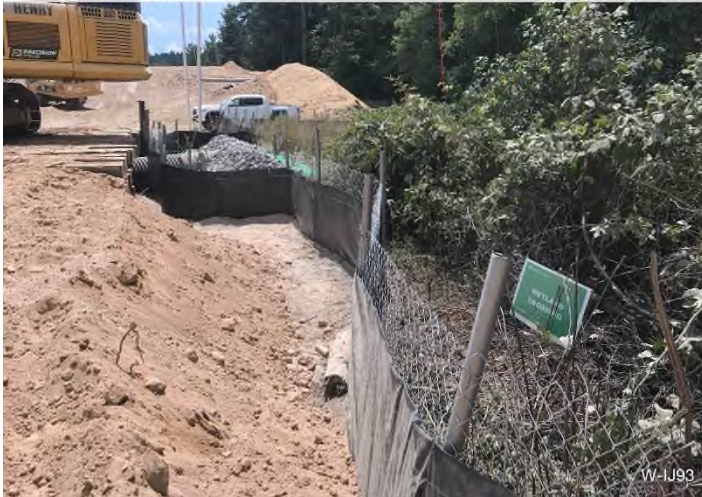
Figure 3: Wetland W-IJ93 – Controls in place and functioning properly.
