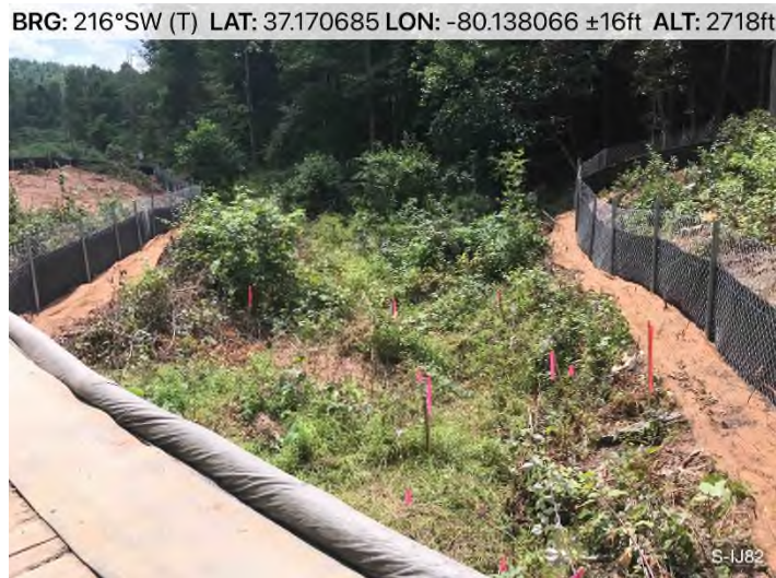
Figure 7: Stream S-IJ82 – Controls in place and functioning properly along stream S-IJ82 crossing.
