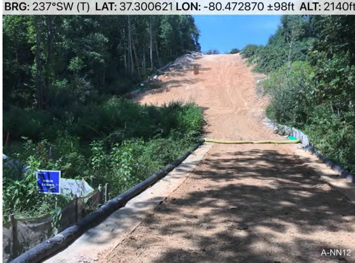
Figure 3: Stream S-NN12 – Controls in place and functioning properly along stream S-NN12. BRG: 237°SW (T) LAT: 37.300621 LON: -80.472870 ±98ft ALT: 2140ft
