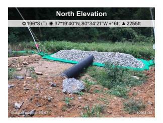
Figure 6: St 10934+80 CWD level spreader lacks perimeter berm and stabilization
