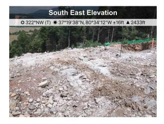
Figure 2: St10967+19 waterbar end treatment appears not to allow water off ROW
