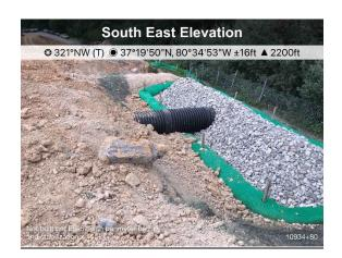
Figure 7: ATWS 1331 fill slope requires rill repair and re stabilization
