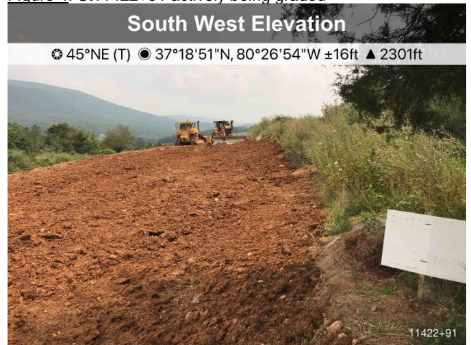
Figure 4: St11422+91 actively being graded
