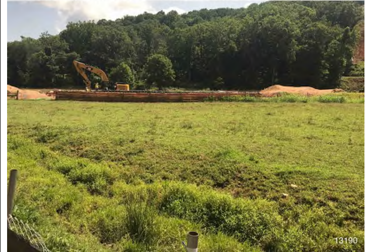
Figure 4: STA 13194+50 – Dewatering structure #1 on west side of the ROW. Discharging onto well vegetated area. No sediment off ROW.
