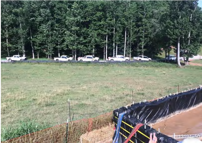
Figure 3: STA 13194+50 – Dewatering structure #1 on west side of the ROW. Discharging onto well vegetated area. No sediment off ROW.
