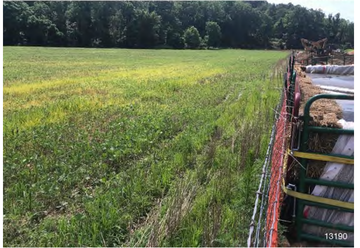
Figure 6: STA 13190+00 – Dewatering structure #2 on east side of the ROW. Discharging onto well vegetated area. No sediment off ROW.
