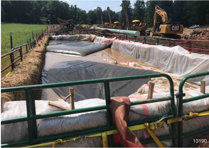
Figure 5: STA 13190+00 – Dewatering structure #2 on east side of the ROW. Pump hoses discharging into sediment bag inside of secondary dewatering structure.
