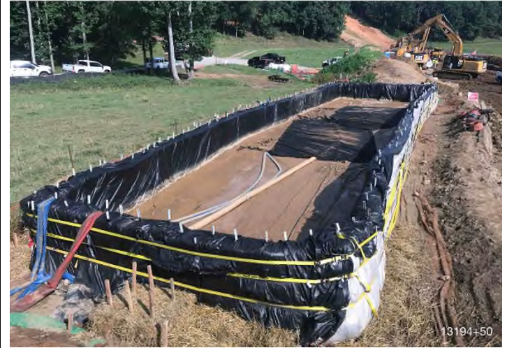
Figure 4: STA 13194+50 – Dewatering structure #1 on west side of the ROW. Discharging onto well vegetated area. No sediment off ROW.
