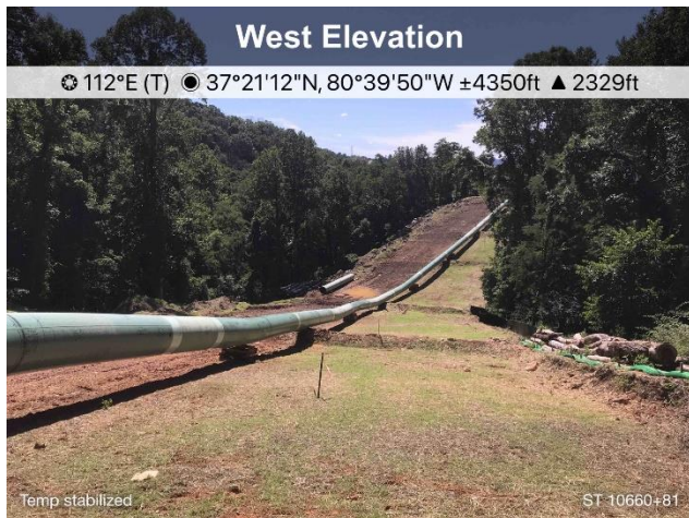
Figure 7: St10660+81 area is temporarily stabilized
