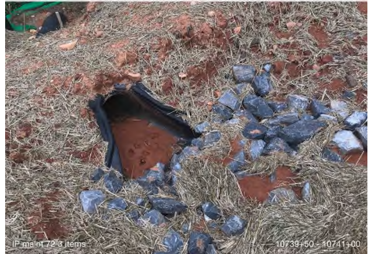
Figure 4: STA 10739+50 to 10741+00 – Inlet protection maintenance needed.
