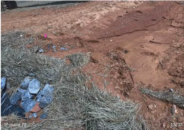
Figure 3: STA 10732+00 – Inlet protection maintenance needed.
