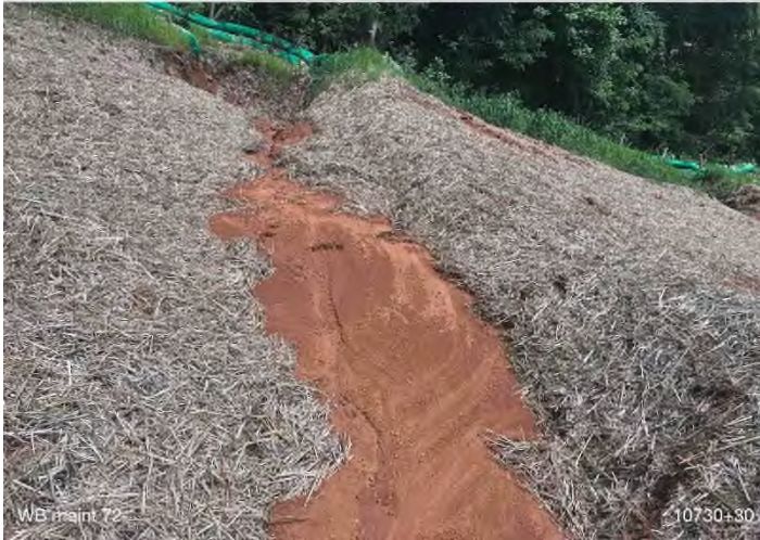
Figure 3: STA 10732+00 – Inlet protection maintenance needed.
