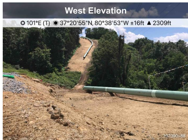
Figure 8: Stabilized area near St10709+88
