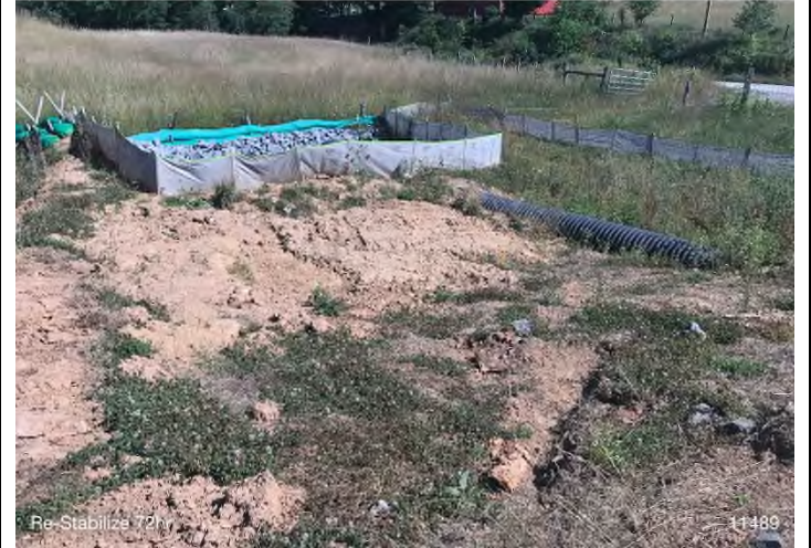
Figure 4: STA 11515+00 – Controls in place and functioning properly. Area stabilized with straw.
