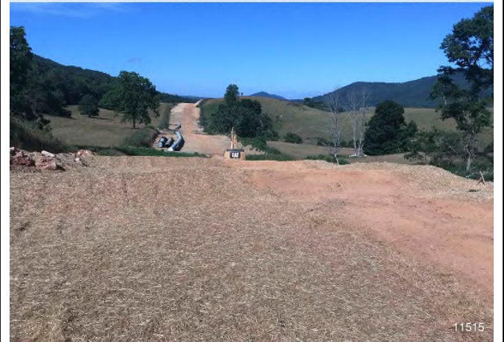
Figure 4: STA 11515+00 – Controls in place and functioning properly. Area stabilized with straw.
