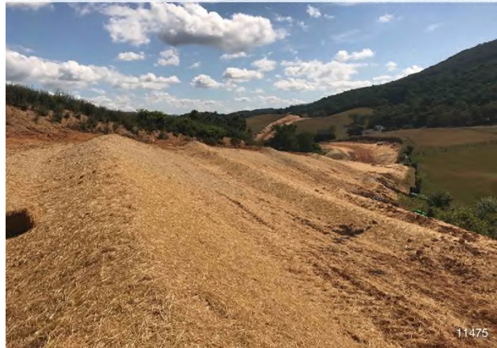
Figure 3: STA 11475+00 – Controls in place and functioning properly. Area stabilized with straw.
