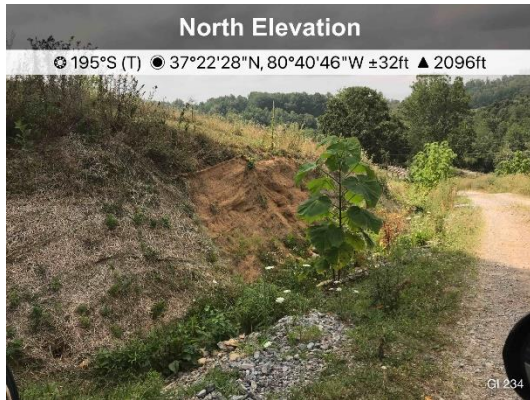
Figure 1: AR GI 234 ditch line
