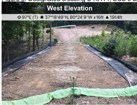
Figure 3: Designated crossing S-RR14, ECD's are in place.
