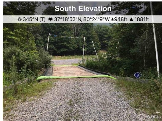
Figure 2: Designated crossing S-RR13, ECD's are in place.
