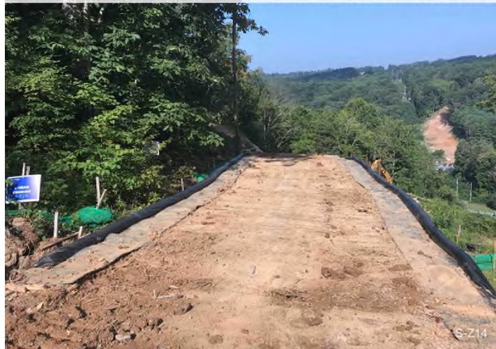
Figure 1: Stream S-Z14 – Controls in place and functioning properly. BRG: 281°W (T) LAT: 37.336314 LON: -80.677131 ±25695ft ALT: 2361ft
