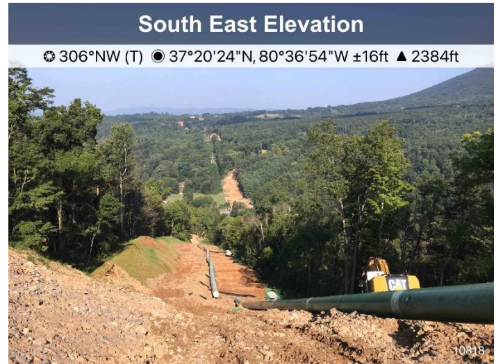
Figure 4: St 10818 ECD ongoing maintenance
