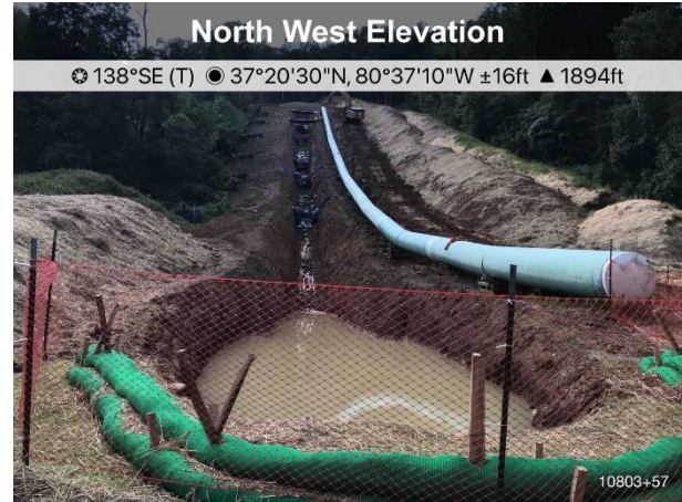
Figure 2: St 10803+57 ECD installed at base of trench.
