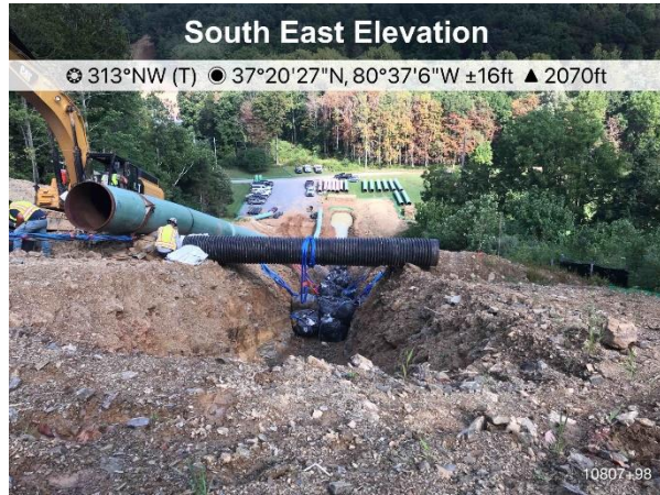
Figure 1: Additional control installed near St 10807+98
