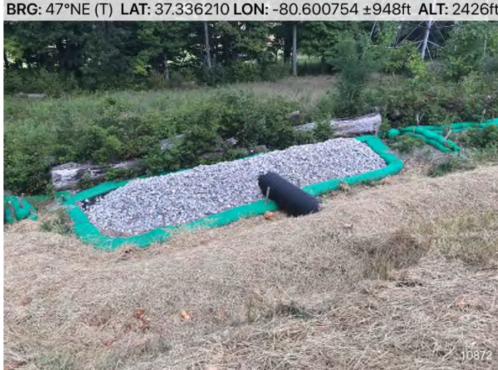
Figure 3: STA 10872+00 – Controls in place and functioning properly. BRG: 47°NE (T) LAT: 37.336210 LON: -80.600754 ±948ft ALT: 2426ft
