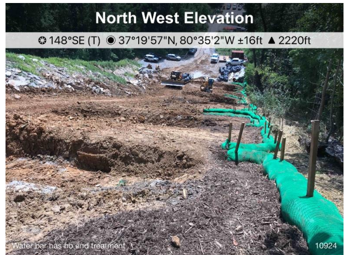
Figure 4: St 10924 waterbar has no end treatment
