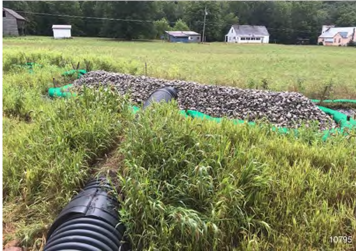
Figure 3: STA 10795+00 – Controls in place and functioning properly.
