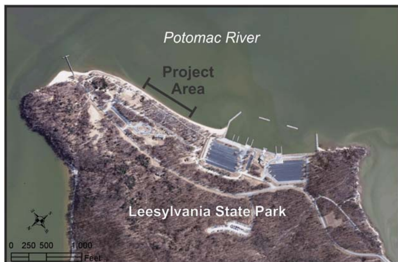
Figure 2. Location of the Living Shoreline sill project at Leesylvania State Park.
