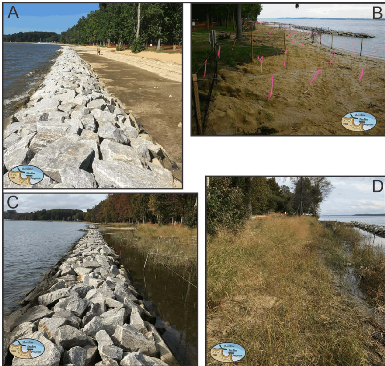
Figure 5. A) Rock sill 1 and sand fill after installation but before marsh planting (12Aug2016); B) Marsh grass planting and goose fence installation (1Sep2016); C) Sill 1 approximately one year after installation (23Oct2017); and D) high marsh grasses behind sill 1 after about one year (23Oct2017). Photos by Shoreline Studies Program, VIMS.
