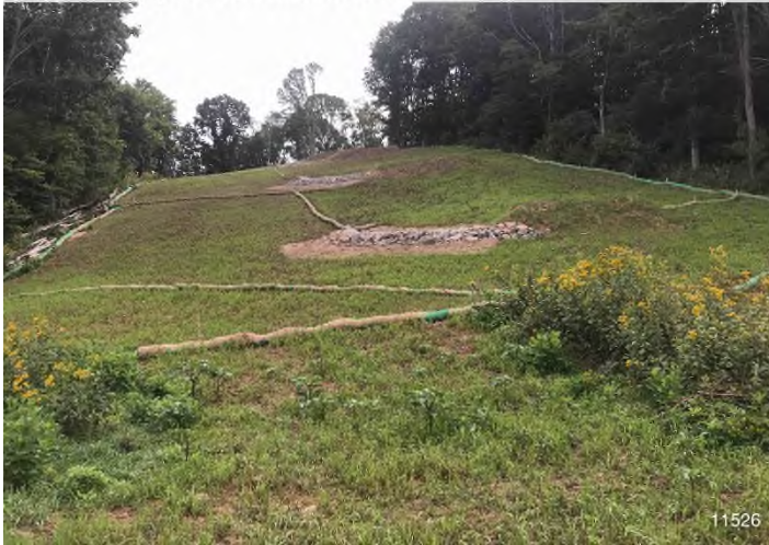
Figure 3: STA 11425+00 – Controls in place and functioning properly.
