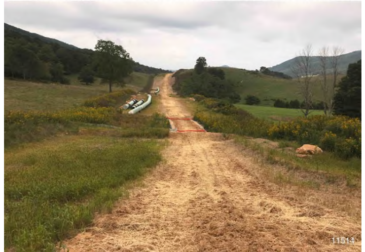
Figure 4: STA 11413+00 – Controls in place and functioning properly.
