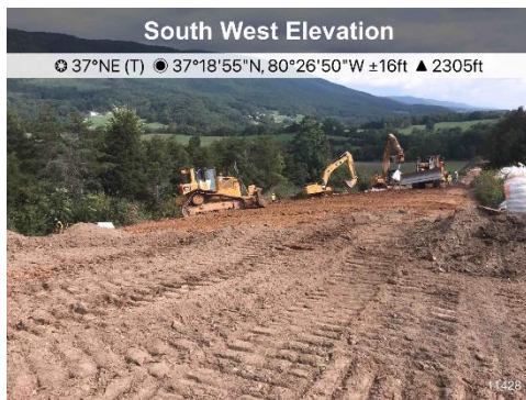
Figure 3: St 11428 on going grading activities and permanent stabilization.
