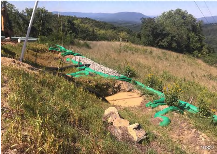
Figure 3: STA 10827+00 – Controls in place and functioning properly.
