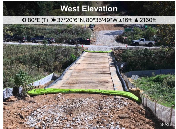
Figure 2: Designated crossing S-A32, ECD's are in place.
