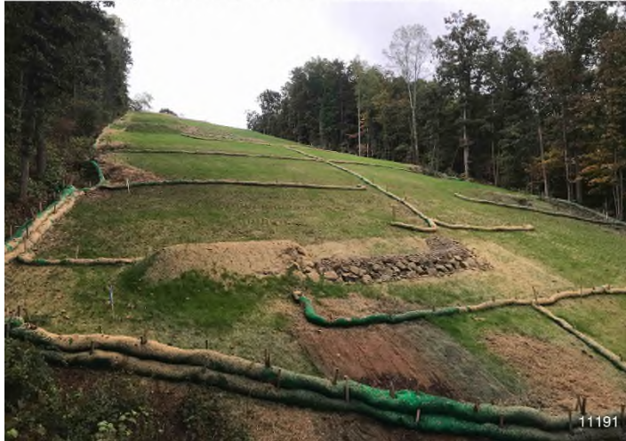
Figure 3: STA 11191+00 – Controls in place and functioning properly. BRG: 111°E (T) LAT: 37.306601 LON: -80.509923 ±98ft ALT: 1720ft
