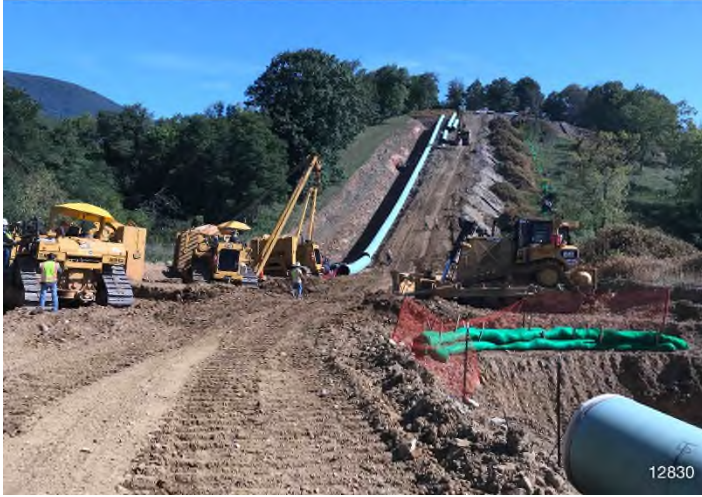
Figure 3: STA 10852+00 – Controls in place and functioning properly.
