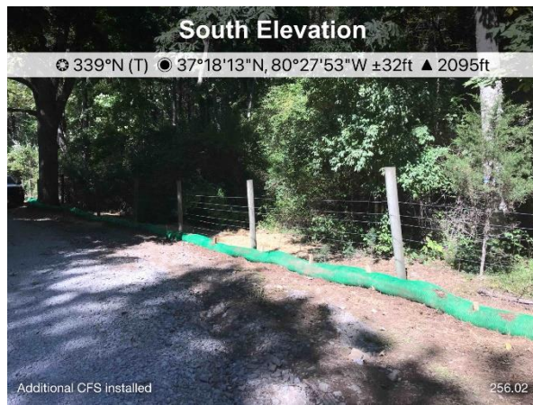
Figure 3: Additional CFS has been installed on portions of AR 256.02.
