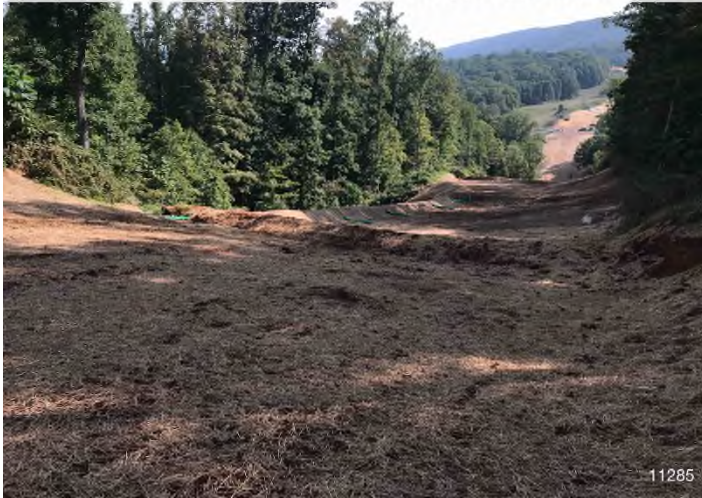
Figure 3: STA 11304+00 – Controls in place and functioning properly. Area stabilized with straw.
