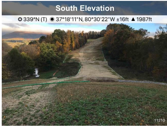
Figure 1: Permanent stabilization and waterbars have been installed near St 11210
