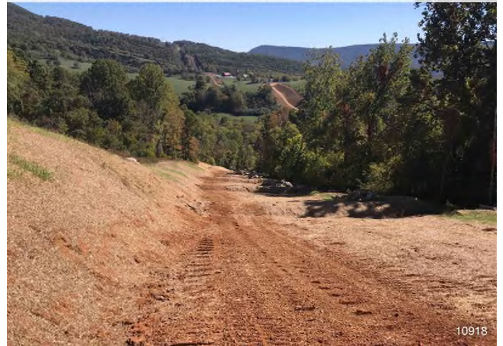
Figure 4: STA 10918+00 – Controls in place and functioning properly. Area stabilized outside of active travel lane. BRG: 131°SE (T) LAT: 37.332882 LON: -80.584734 ±213ft ALT: 2233ft
