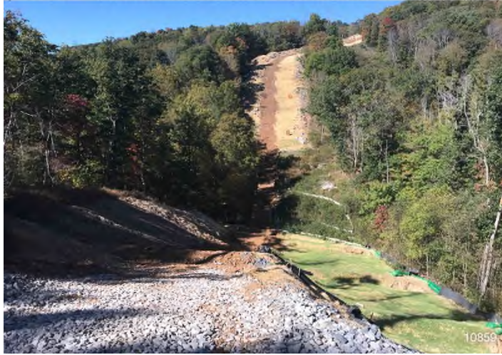
Figure 1: STA 10859+00 – Controls in place and functioning properly. Area stabilized outside of active travel lane. BRG: 291°W (T) LAT: 37.337672 LON: -80.604354 ±98ft ALT: 2288ft
