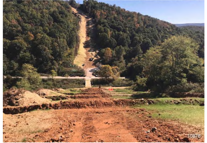
Figure 2: STA 10878+00 – Controls in place and functioning properly. Area stabilized outside of active travel lane. BRG: 89°E (T) LAT: 37.335681 LON: -80.598313 ±16ft ALT: 2296ft
