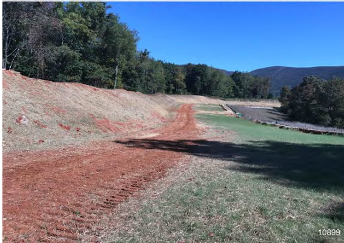
Figure 3: STA 10899+00 – Controls in place and functioning properly. Area stabilized outside of active travel lane. BRG: 11°N (T) LAT: 37.334599 LON: -80.592117 ±98ft ALT: 2540ft
