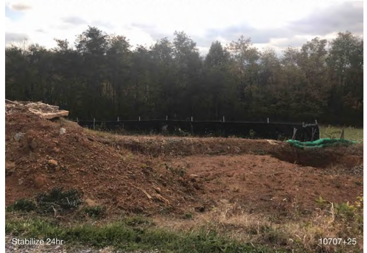
Figure 4: STA 10728+00 – Controls in place and functioning properly. Area stabilized with straw.
