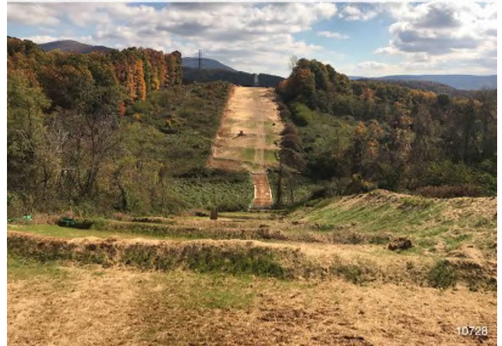
Figure 4: STA 10728+00 – Controls in place and functioning properly. Area stabilized with straw.
