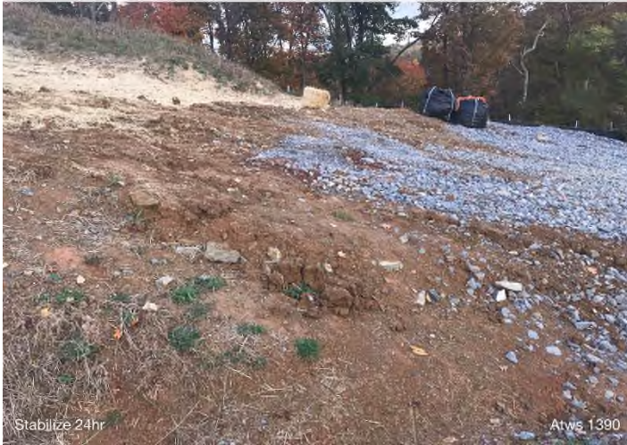
Figure 3: STA 10676+15 –Stabilization needed.
