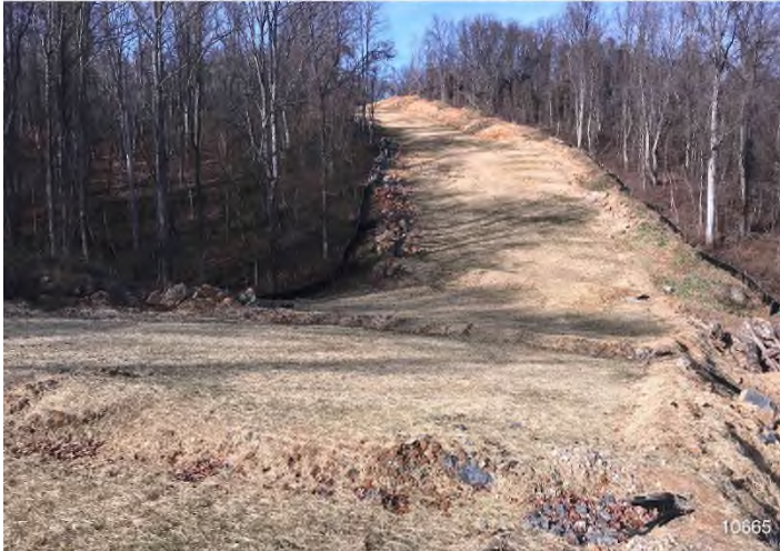
Figure 3: STA 10665+00 – Controls in place and functioning properly. Area stabilized with straw
