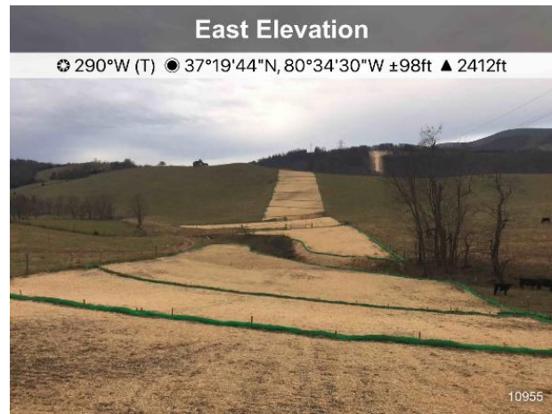
Figure 4: St10955 area has been stabilized and ECD's are in place.
