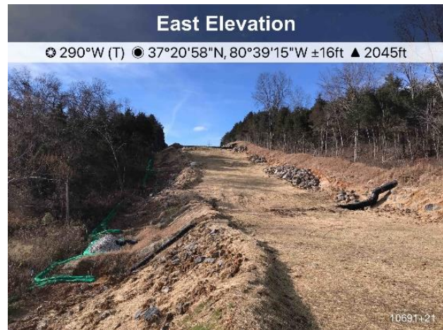
Figure 4. St10691+21 ECD's are in place.
