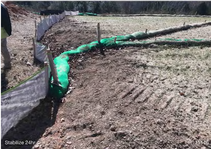
Figure 3: STA 11146+15 –Stabilization needed.
