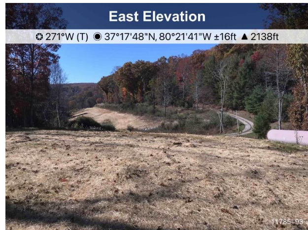
Figure 4: St11785+93 ECD's are in place and area is stabilized.
