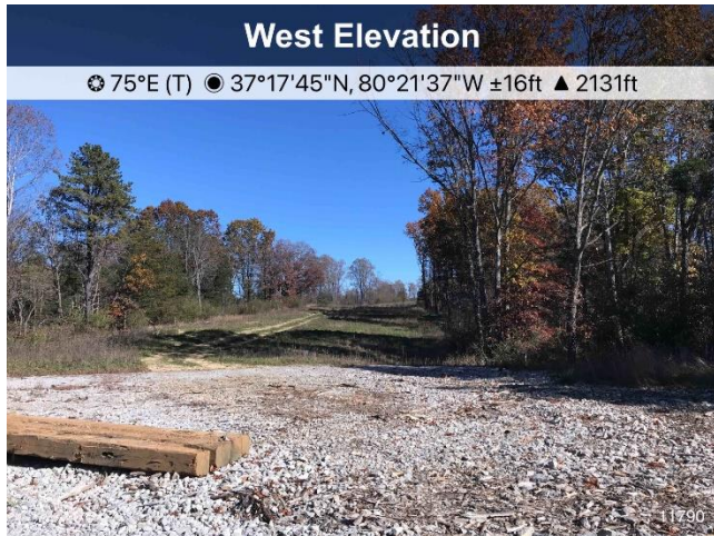
Figure 1: St11790 area is stabilized and ECD's are in place.
