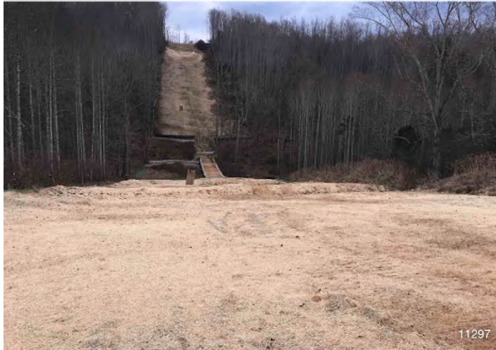
Figure 1: STA 11297+00 – Controls in place and functioning properly. Area stabilized with straw BRG: 259°W (T) LAT: 37.296326 LON: -80.479501 ±164ft ALT: 1950ft
