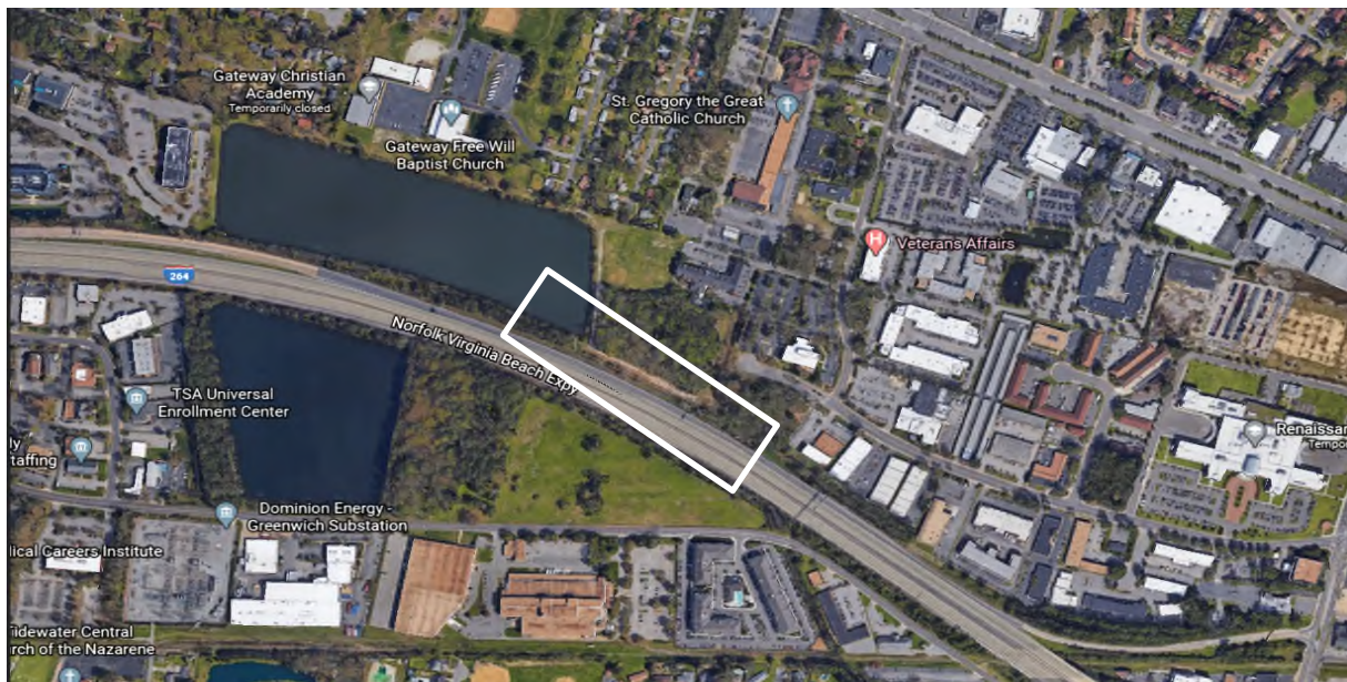
Figure 4 Overhead of WB I-264 between Newtown Road and Witchduck Road
