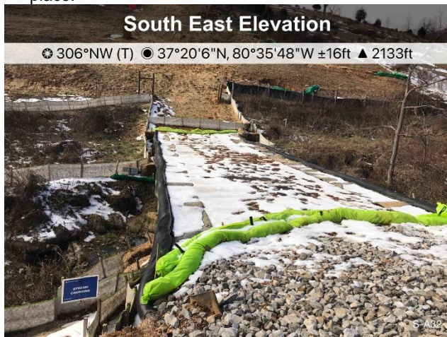
Figure 3: Designated stream crossing S-A32, ESC controls were in place.
