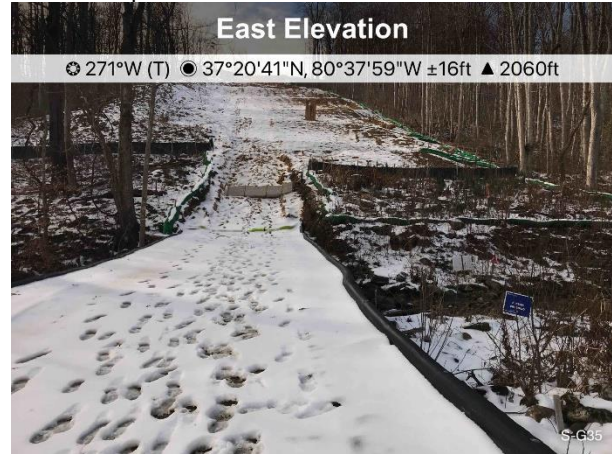
Figure 2: Designated stream crossing S-G35, ESC controls were in place.
