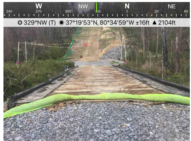
Figure 4: Designated crossing S-Y3, ESC's are in place and functioning.
