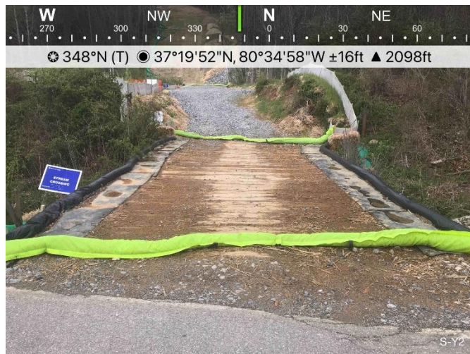
Figure 3: Designated crossing S-Y2, ESC's are in place and functioning.
