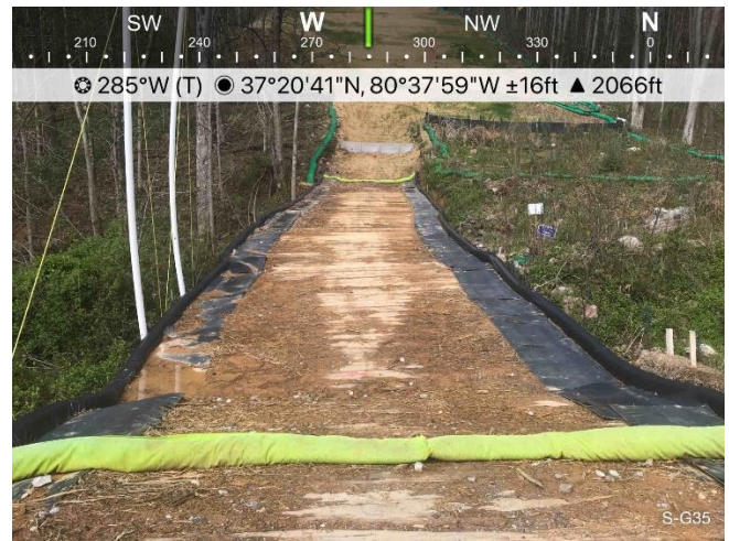
Figure 2: Designated crossing S-G35, ESC's are in place and functioning.
