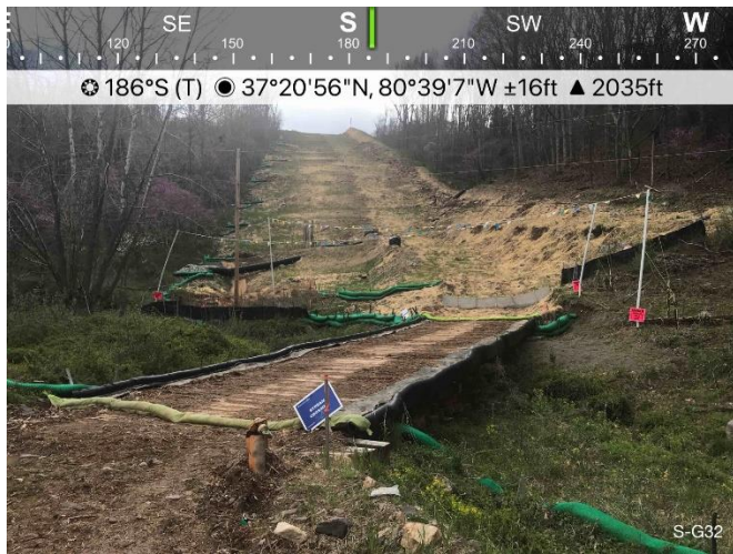
Figure 1: Designated crossing S-G32, ESC's are in place and functioning.
