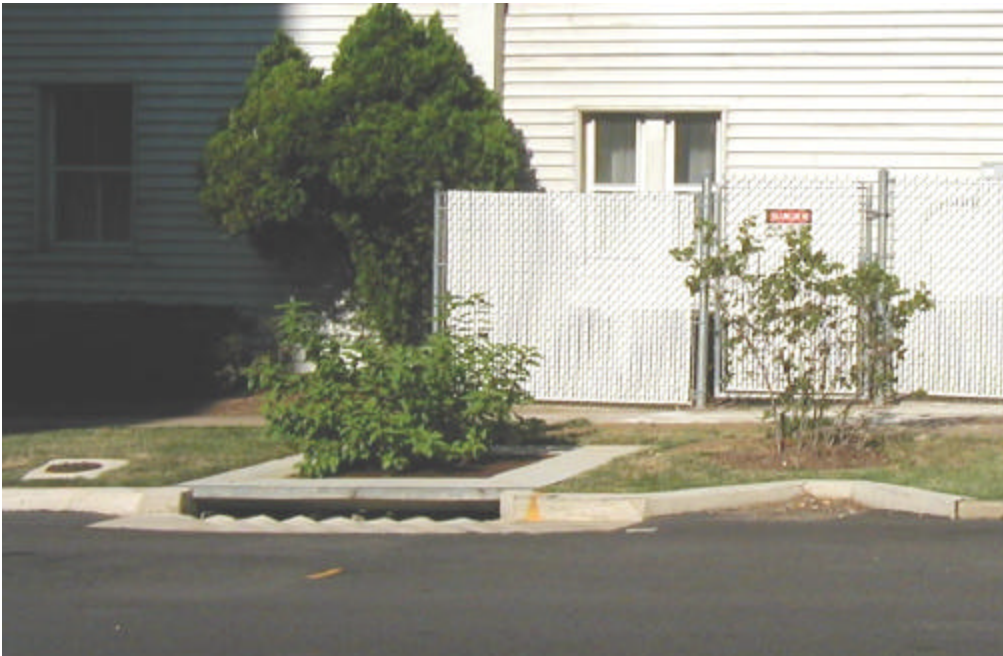
Figure 1. Filtterra™ Urban Streetscape Design
