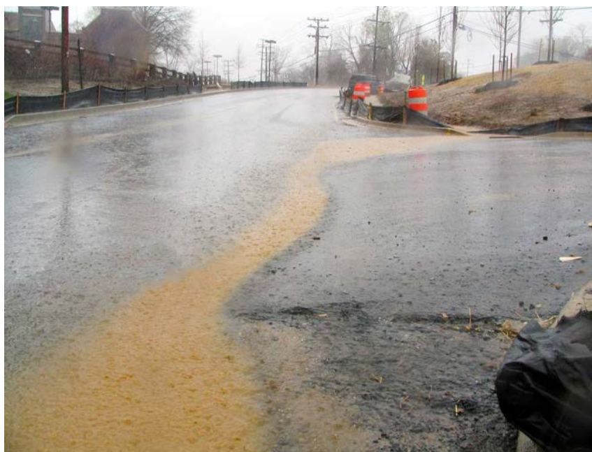
Figure 4.33 Construction Site Erosion
