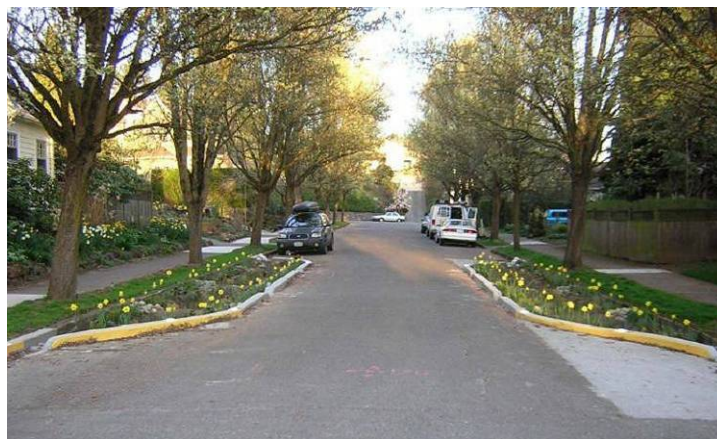
Figure 5-C.21. A Neighborhood Green Street Retrofit Project Source: Chesapeake Bay Stormwater Training Partnership
