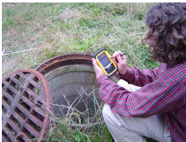
Figure 5-D.25. Storm Drain Inlet Inspection
