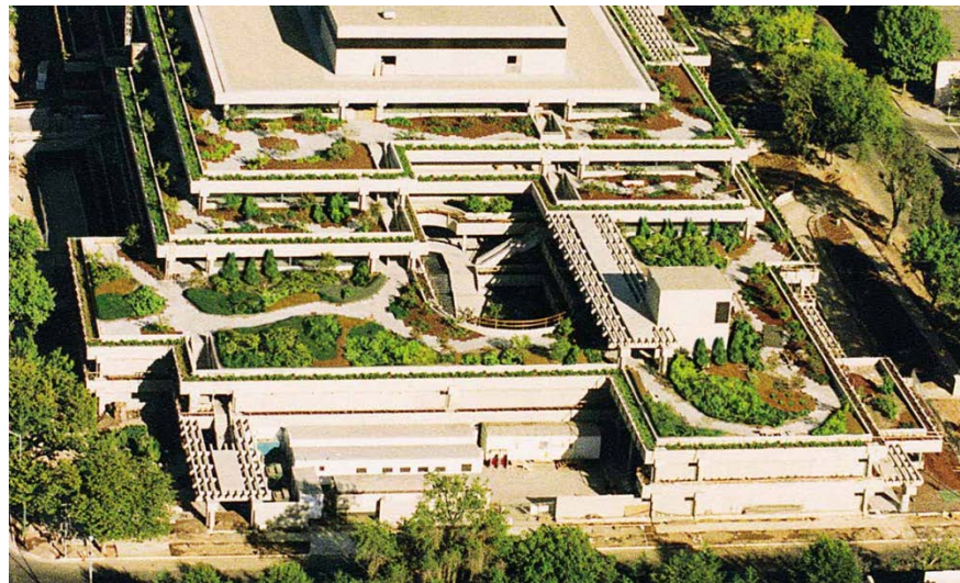
Figure 5-C.11. Vegetated Roofs in an Urban Area Source: Chesapeake Bay Stormwater Training Partnership
