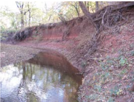
Figure 5-B.7. Streambank erosion along the Little River
