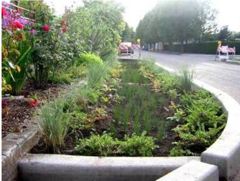
Figure 5-C.17. Bioretention Along a Green Street
