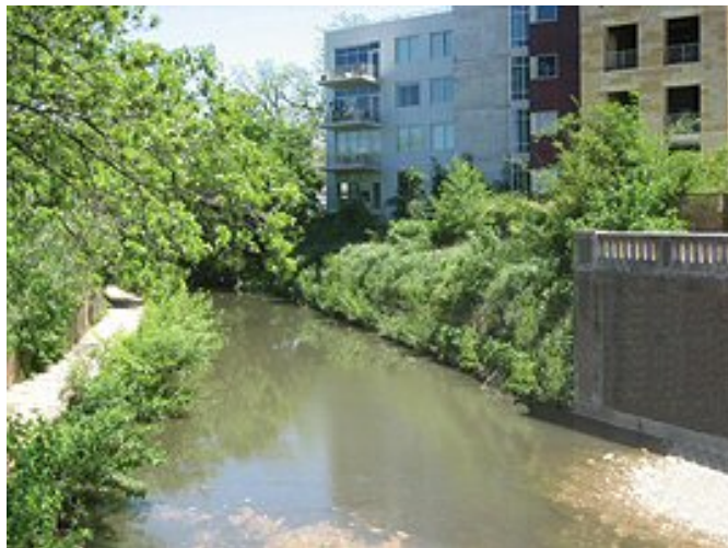
Figure 5-B.9. This reach of Shoal Creek was restored Using bioengineered techniques and natural materials
