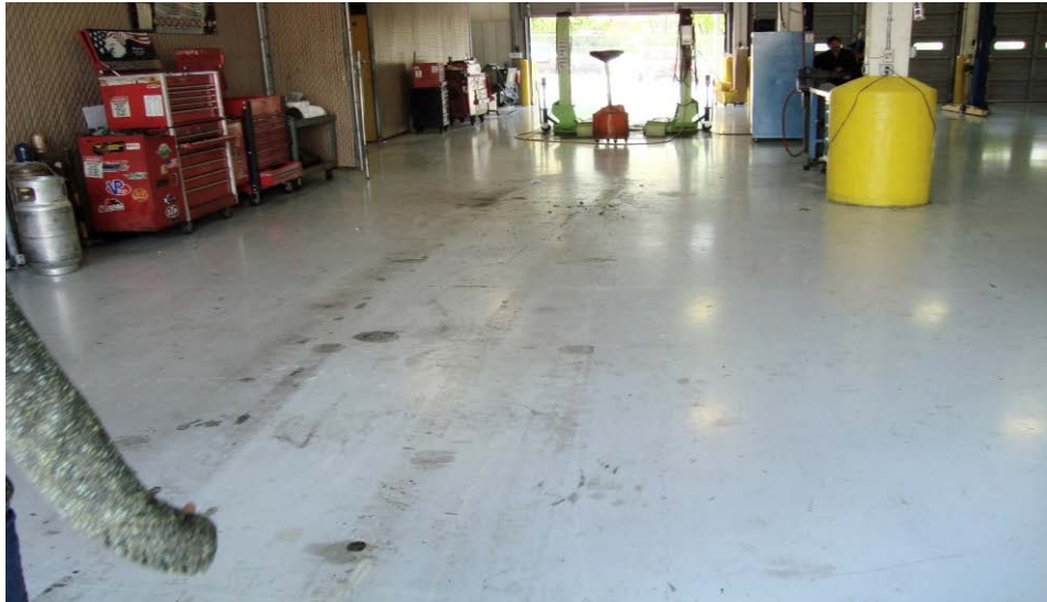
Figure 5-D.12. Indoor Truck Maintenance Area (with Proper Storage for Used Fluids, Rags, Solvents and Other Materials)
