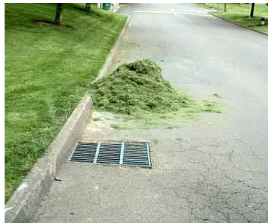
Figure 5-D.21. Lawn Clippings Left Along the Curb Can Be Washed Into the Storm Drain
