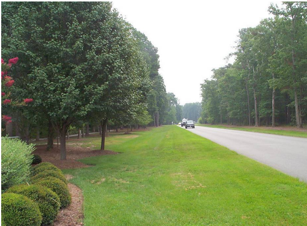
Figure 6.87. Dry swale along a suburban connector street (no curb and gutter). Source: Chesapeake Bay Stormwater Training Partnership
