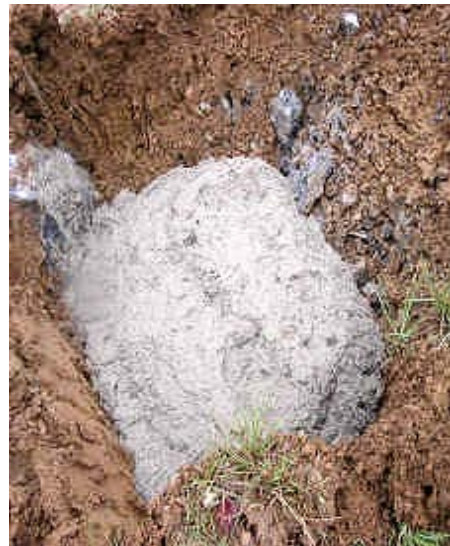
Figure 6-B.23. Grouting a Sinkhole
