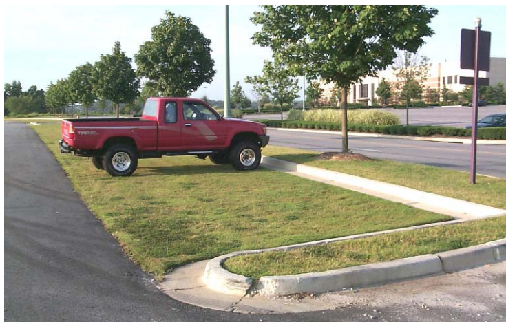
Figure 6.62. Grass Paver Surface Used for Parking Source: ARC (2001)
