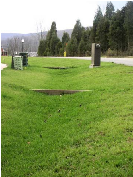
Figure 6.91. Grass Channel in Median.
