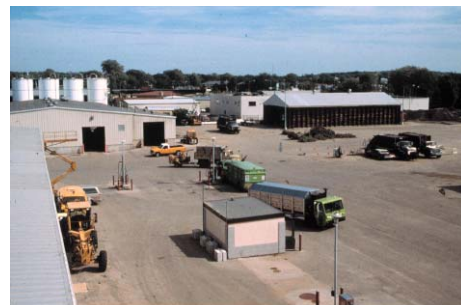
Figure 6.124. Public Works Yard
