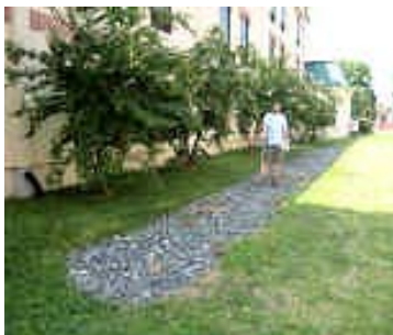
Figure 6-B.19. Small-Scale Infiltration Trench
