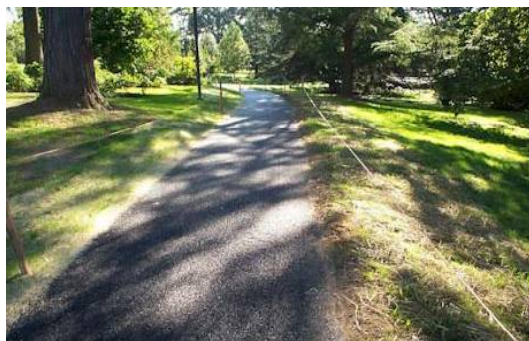
Figure 6.99. Porous Asphalt Bike Path
