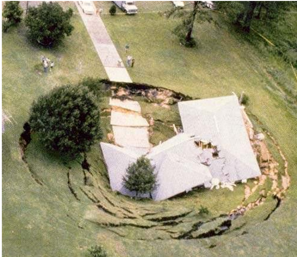
Figure 6-B.4. A House Destroyed by a Sinkhole.
