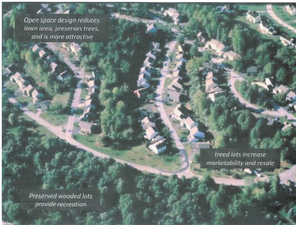
Figure 6.43. Aerial View of an Open Space Subdivision Source: Chesapeake Bay Stormwater Training Partnership
