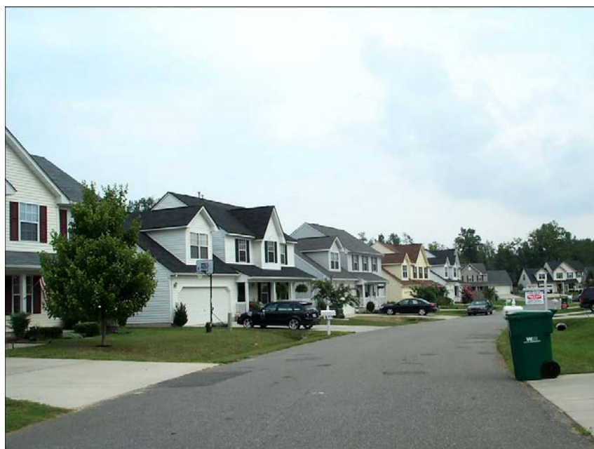
Figure 6.46. Narrow Residential Street with Swale Drainage Source: Chesapeake Bay Stormwater Training Partnership
