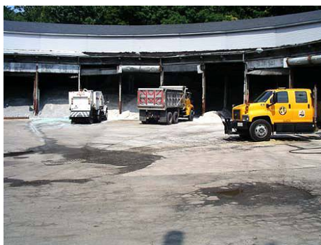
Figure 6.126. Covered Chemical Storage
