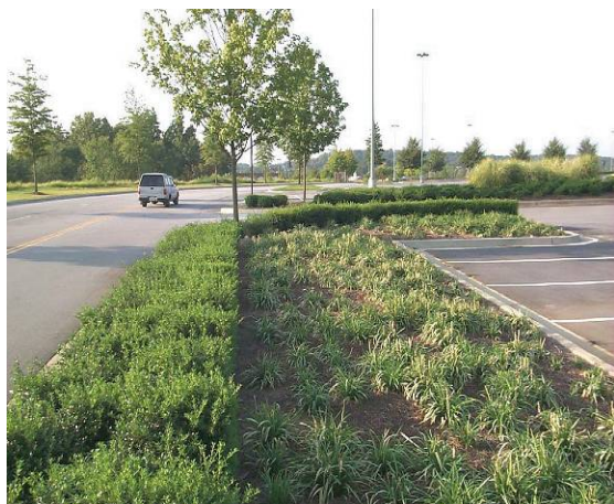
Figure 6.76. Parking Lot Stormwater Island
