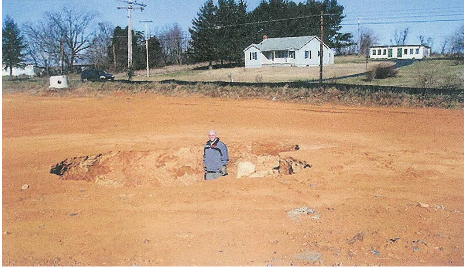
Figure 6-B.8. Sinkhole at a Construction Site
