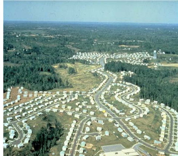
Figure 6.16. Subdivision Cleared and Grubbed from Property Line to Property Line
