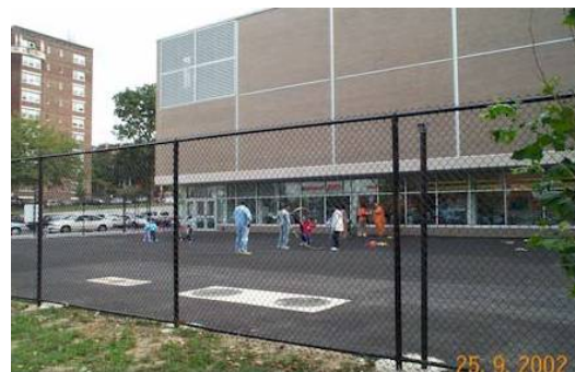
Figure 6.100. Porous Asphalt Playing Court
