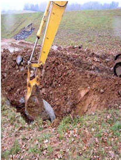
Figure 6-B.22. Sinkhole Remediation
