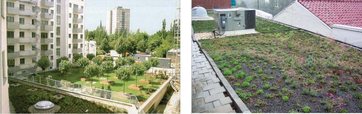
Figure 7.40. Green rooftops can also treat the quality of runoff from flat rooftops. Source: CWP, 2007a
