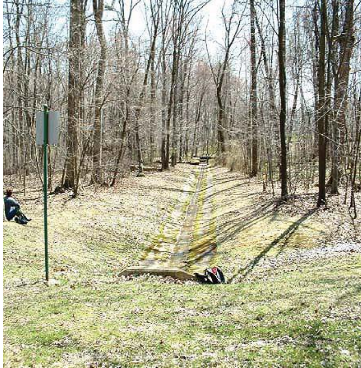
Figure 7.14. Example of a “cutoff” outfall discharging well away from the stream to a wetland area (out of picture) Source: CWP, 2007
