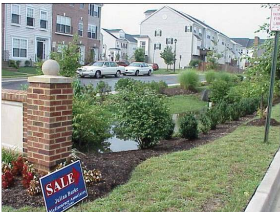
Figure 7.24. Bioretention in Street Median Source: CWP, 2007a
