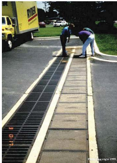
Figure 7.35. Filtering Practices Are Preferred for Retrofits at Hotspot Sites. Source: CWP, 2007a
