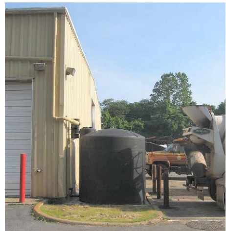
Figure 7-A.19. City Yard Cistern Retrofit
