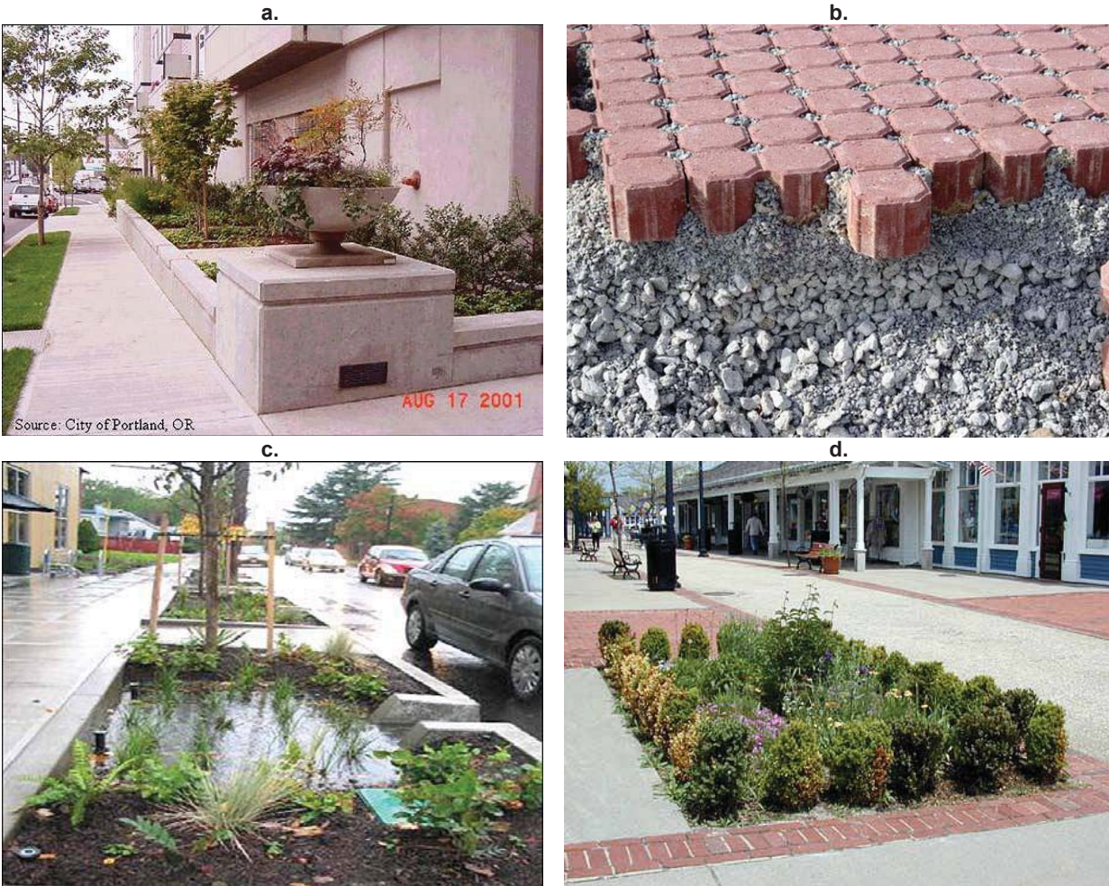
Figure 7.43. Landscape architects can creatively use stormwater as a resource in (a) foundation planters; (b) permeable pavers; (c) bioretention; and (d) stormwater tree pits. Source: CWP, 2007a
