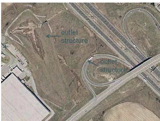
Figure 7.21. Highway retrofits really stand out in aerial photos, although highway drainage does not. Source: CWP, 2007
