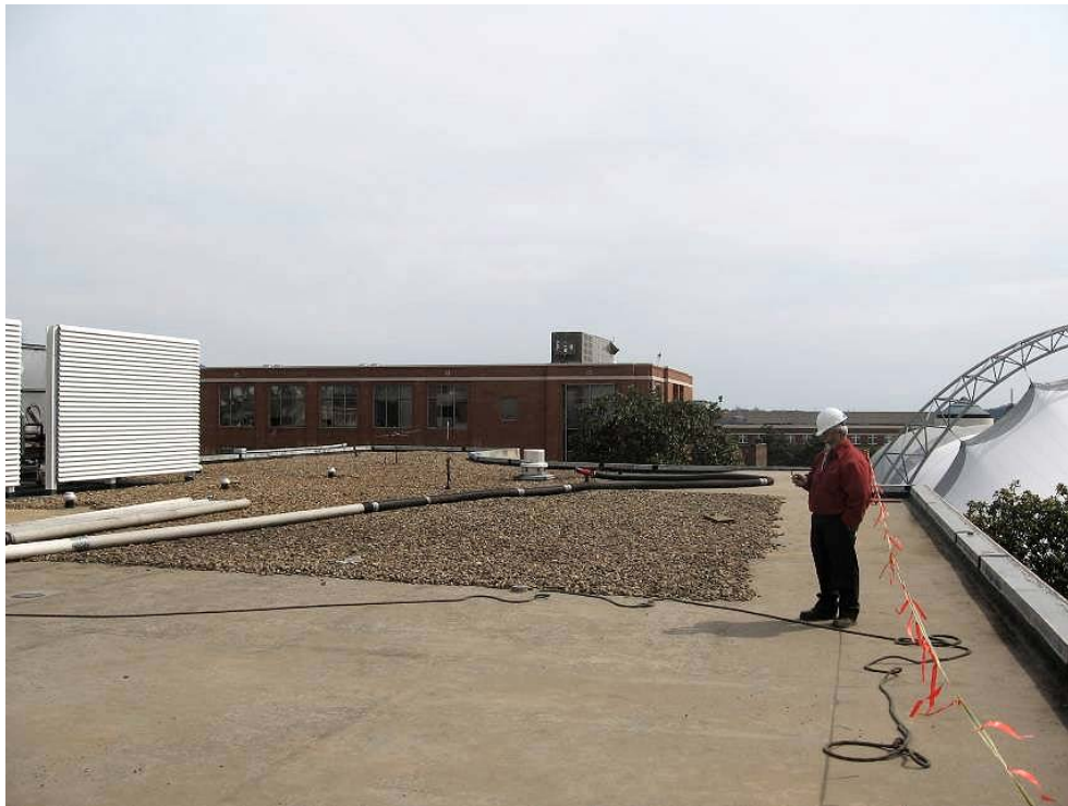
Figure 7-A.16. Original Roof on City Hall
