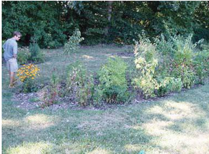
Figure 7.41. Rain Garden Treating Runoff from a Trail
