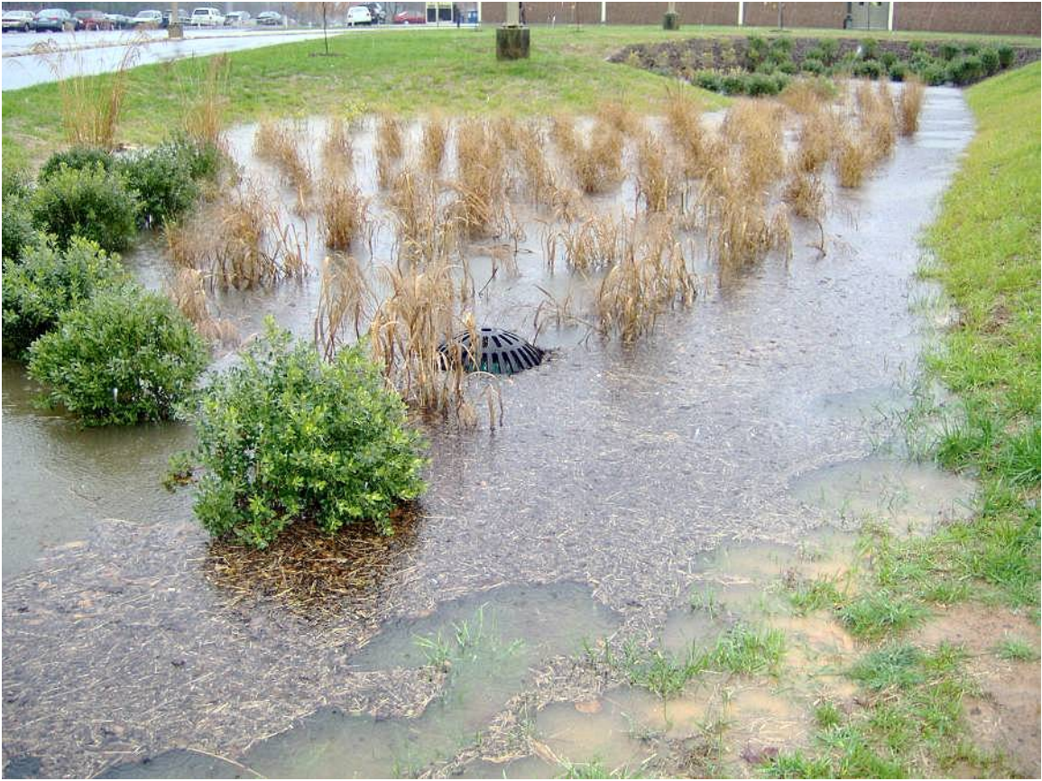
Figure 7-A.13. Charlottesville High School Bioretention Filter
