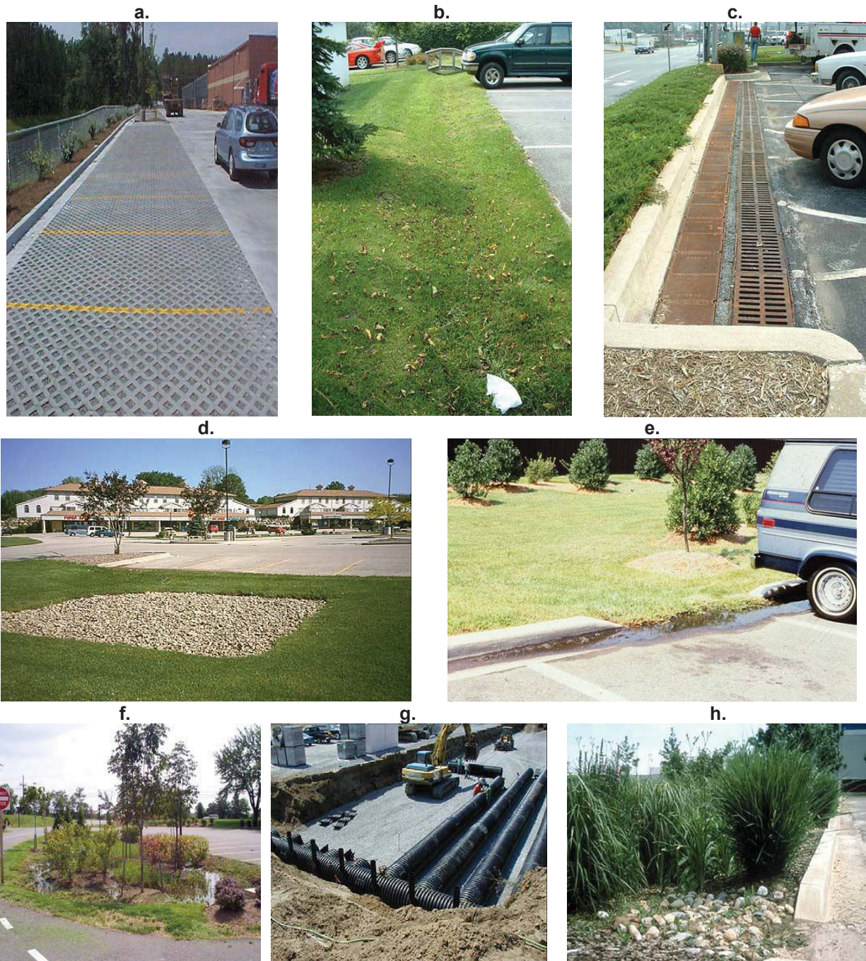
Figure 7.33. Examples of retrofits employed at small parking lots: (a) permeable pavers; (b) dry swale; (c) perimeter sand filter; (d) grass filter/infiltration trench; (e) filter strip; (f) internal bioretention; (g) underground infiltration; and (h) island bioretention. Source: CWP, 2007a
