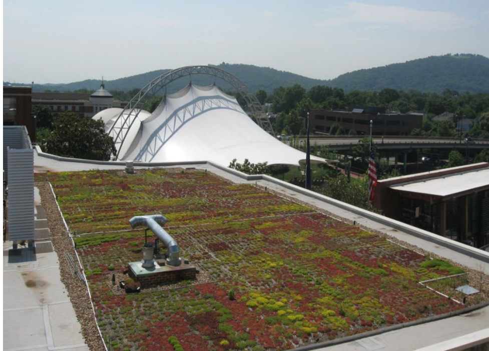
Figure 7-A.17. Replacement Vegetated Roof Area on City Hall
