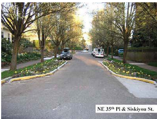
Figure 7.26. Bioretention in Traffic Calming Areas. Source: CWP, 2007a
