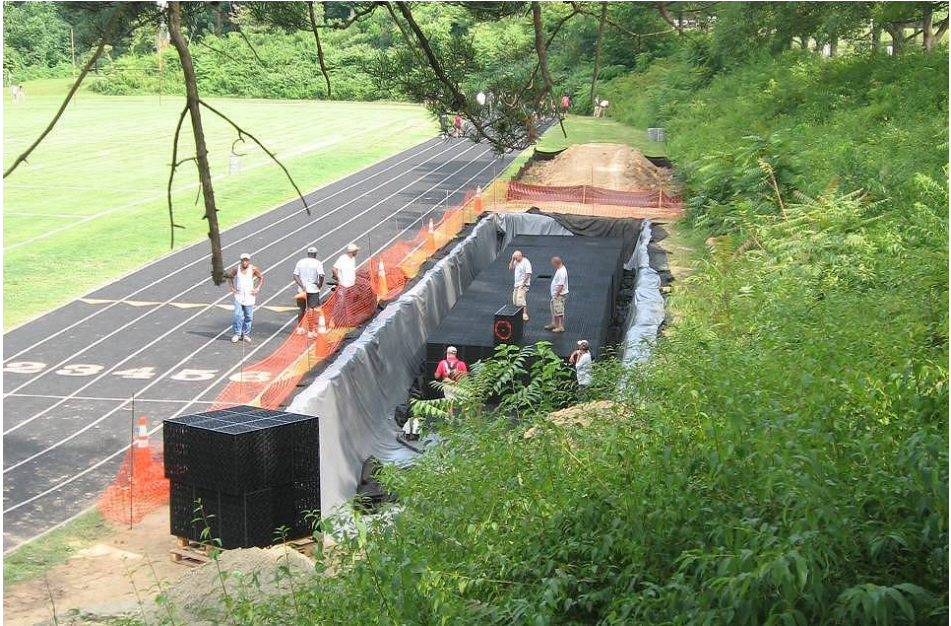
Figure 7-A.11. Construction of the Underground Rainwater Harvesting Cistern at the High School
