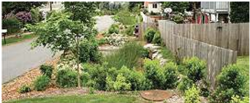
Figure 7.4. Finished Swale Cells Along Seattle's 107 th Street, an East-West Street. Source: Aird, 2009
