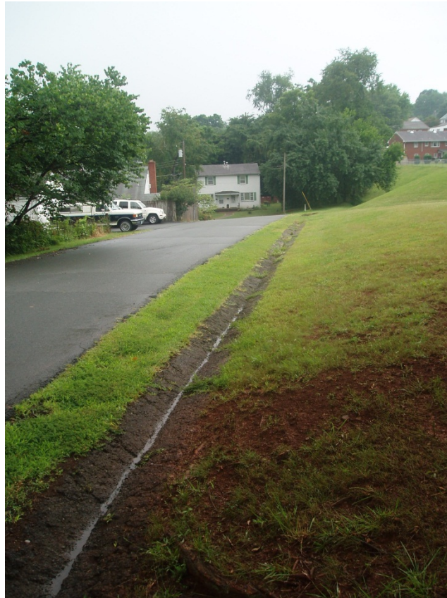
Figure 7-A.12. Existing Asphalt Swale to be Converted
