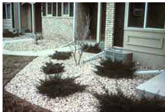
Figure 8.27. Downspout Disconnection
