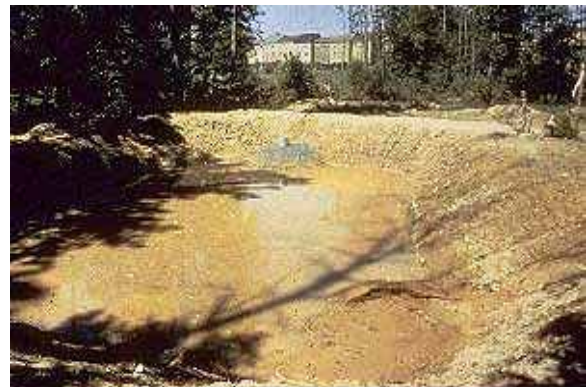
Figure 8.2. Temporary Sediment Basin
