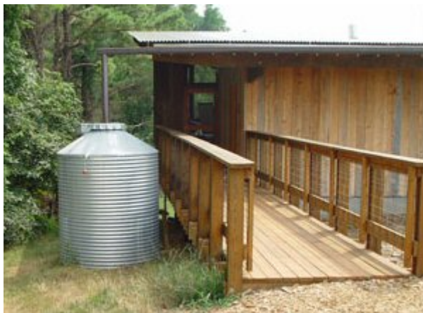
Figure 8.28.. Rainwater Harvesting Tank
