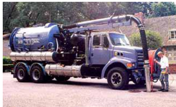
Figure 8.24. Catch Basin Cleaning
