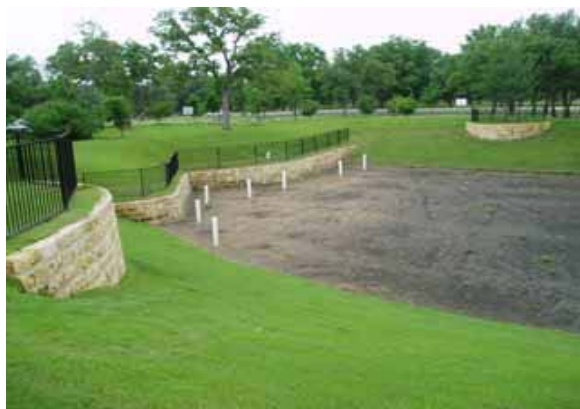
Figure 8.17. Austin Sand Filter
