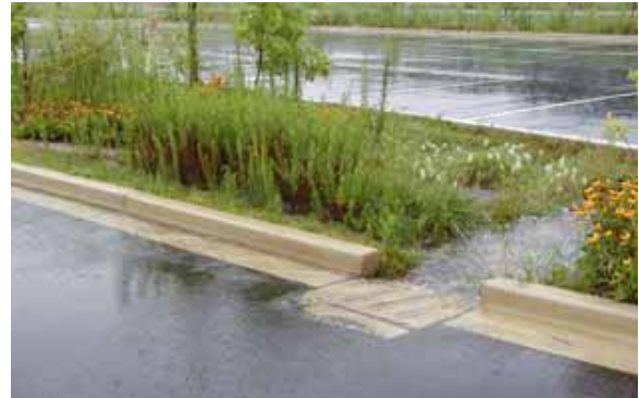
Figure 8.6. Parking Area Bioretention
