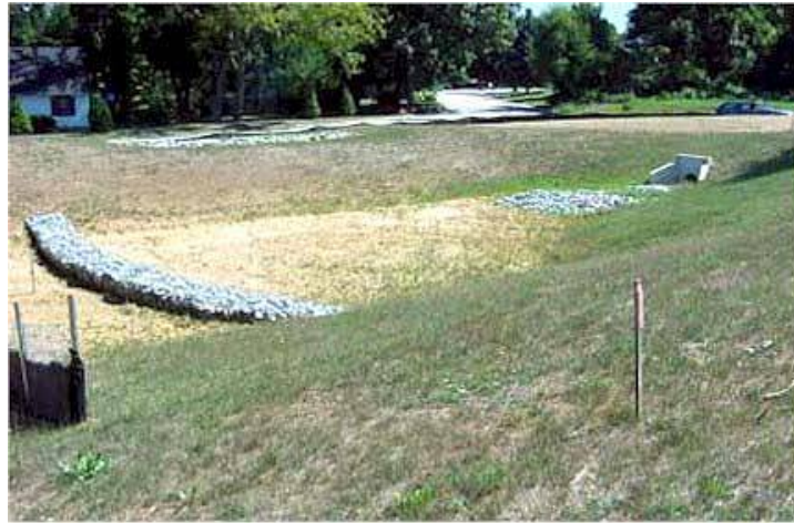
Figure 8.40. Dry Extended Detention Basin
