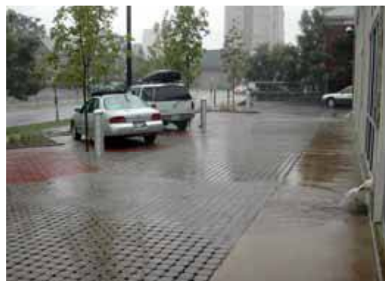
Figure 8.12. Interlocking Permeable Pavers
