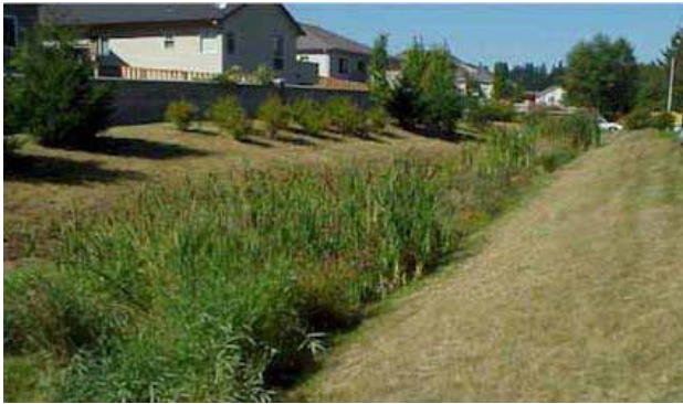
Figure 8.5. Vegetated Wet Swale
