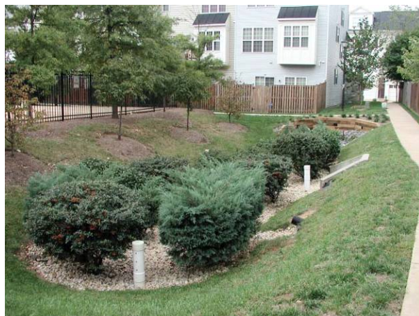
Figure 8.33. Bioretention Filter Cell
