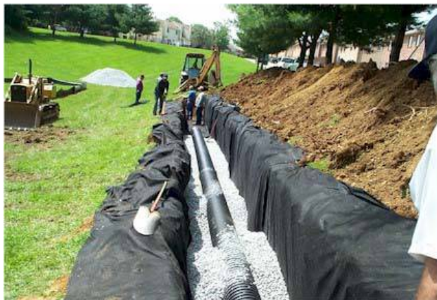
Figure 8.36. Infiltration Trench Construction
