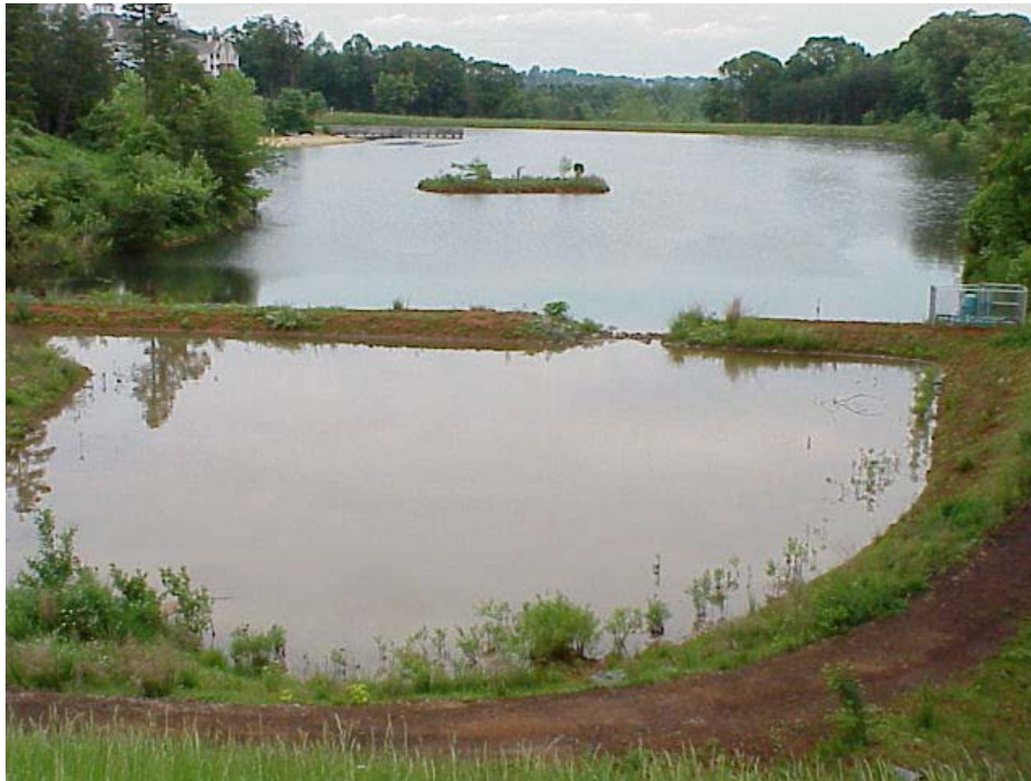
Figure 8.16. Sediment Forebay, with Wet Pond in the Background
