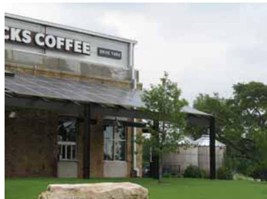
Figure 8.4 Above-Ground Rain Tanks
