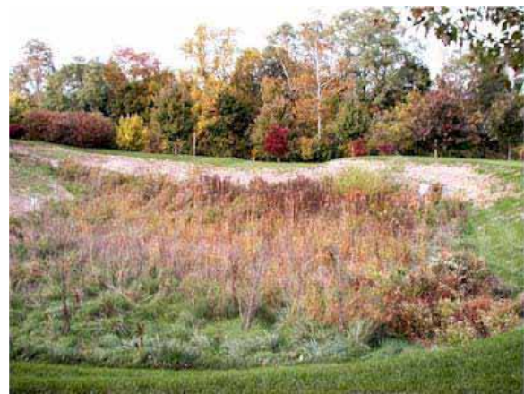
Figure 8.15. Dry Extended Detention Basin
