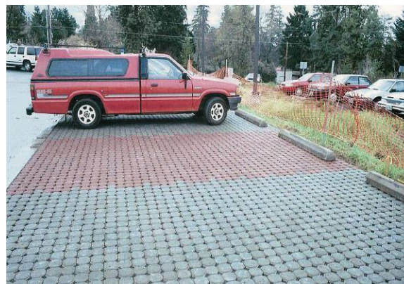
Figure 8.35. Permeable Interlocking Pavers
