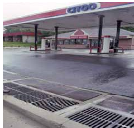
Figure 8.18. Delaware Sand Filter
