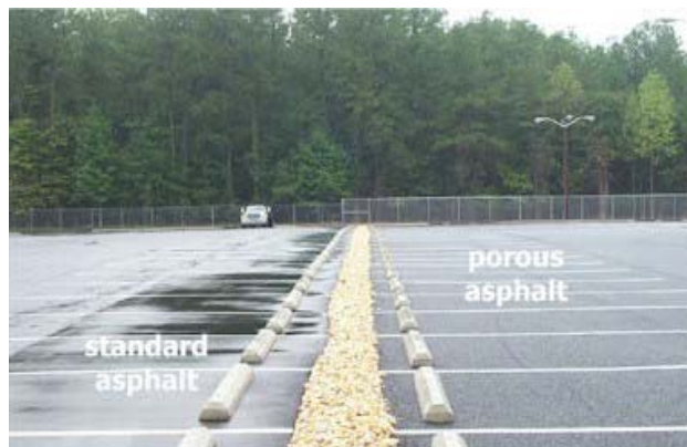
Figure 8.34. Permeable Asphalt Pavement
