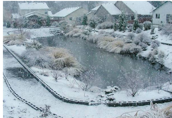
Figure 8.39. Small Wet Pond
