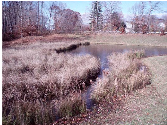
Maintenance Access and Safety: Shallow side slopes and wetland benches Are a maintenance and safety feature.
