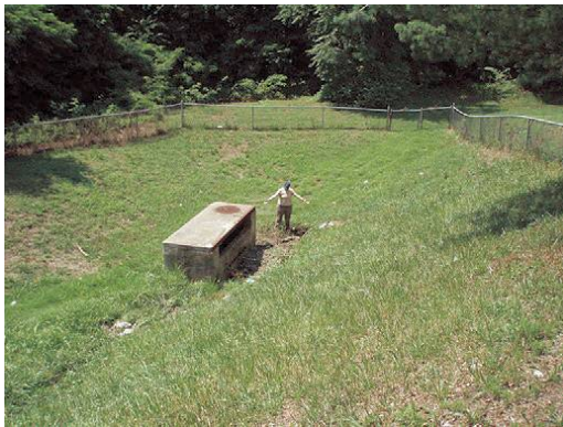
No Planting Plan: Lack of plants and landscaping make BMPs Unattractive and undesirable to maintain.
