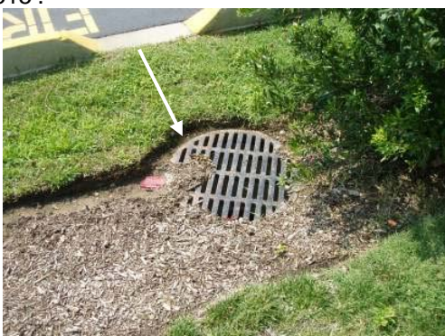
Figure 9-D.3. Examples of Improper BMP Design (Source: CWP, 2009)
