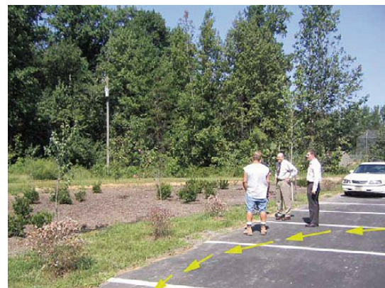
Some site runoff bypasses bioretention.
