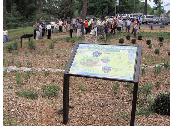
Community Amenity: Stormwater BMPs, such as this rain garden, can be Designed as amenities, with plantings, interpretive Signage, and public access.
