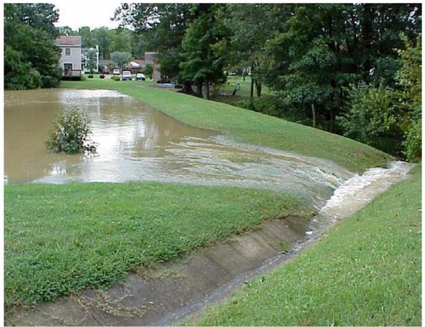
Figure C-2. Emergency Spillway Draining into a Concrete Channel [NOTE: Not sure how appropriate this photo is, since this Appendix focuses on vegetated emergency spillways and does not address this type of design. Perhaps we should delete this photo?]
