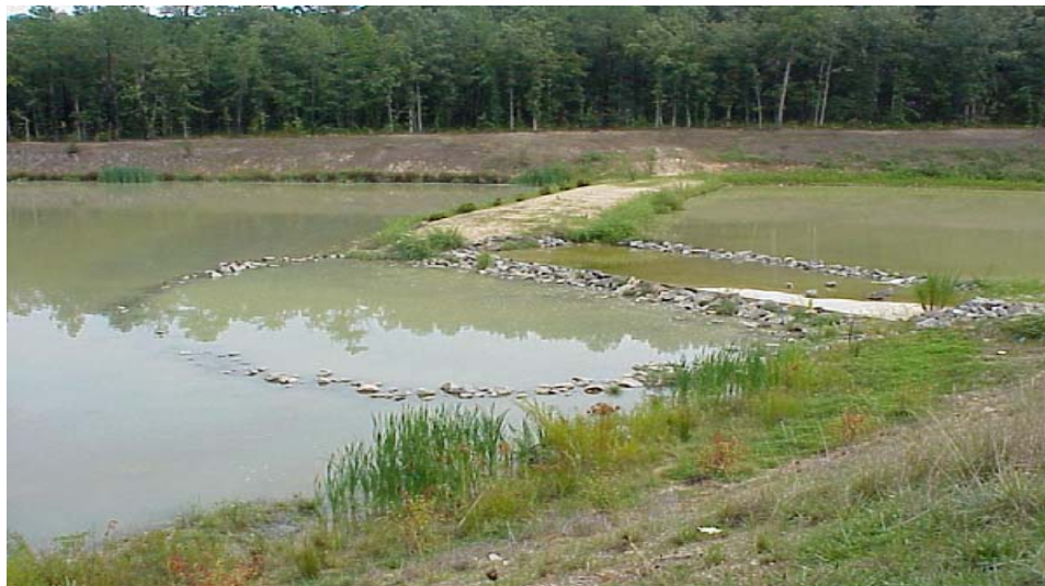
Figure D-3. Sediment Forebay Constructed with a Submerged Rip-Rap Weir
