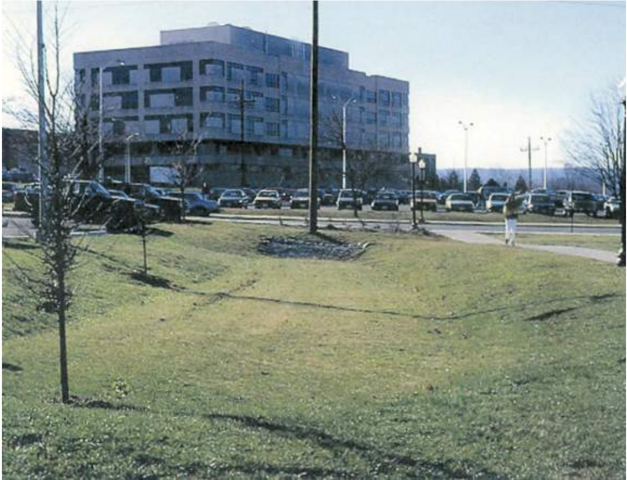
Figure 10.1. Typical Dry Swale in commercial/office setting
