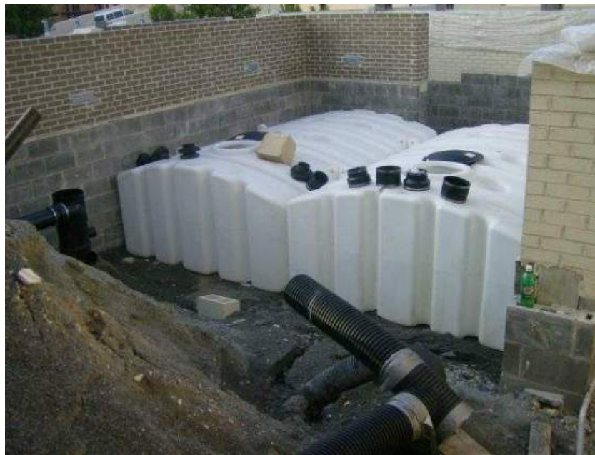
Figure 6.13. Example of two Polyethylene Cisterns
