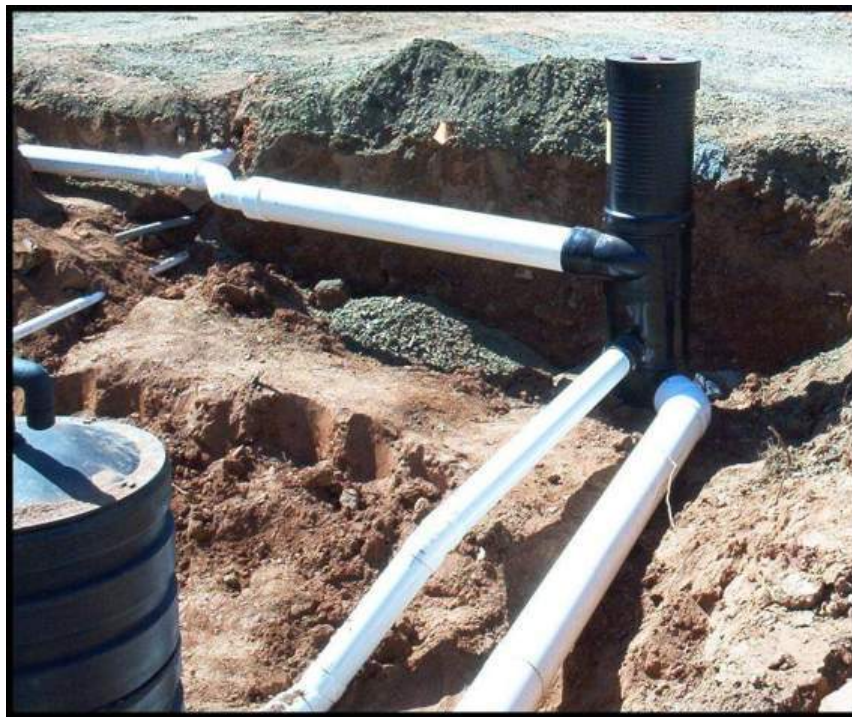
Figure 6.11. Installation of Vortex Filter prior to backfill
