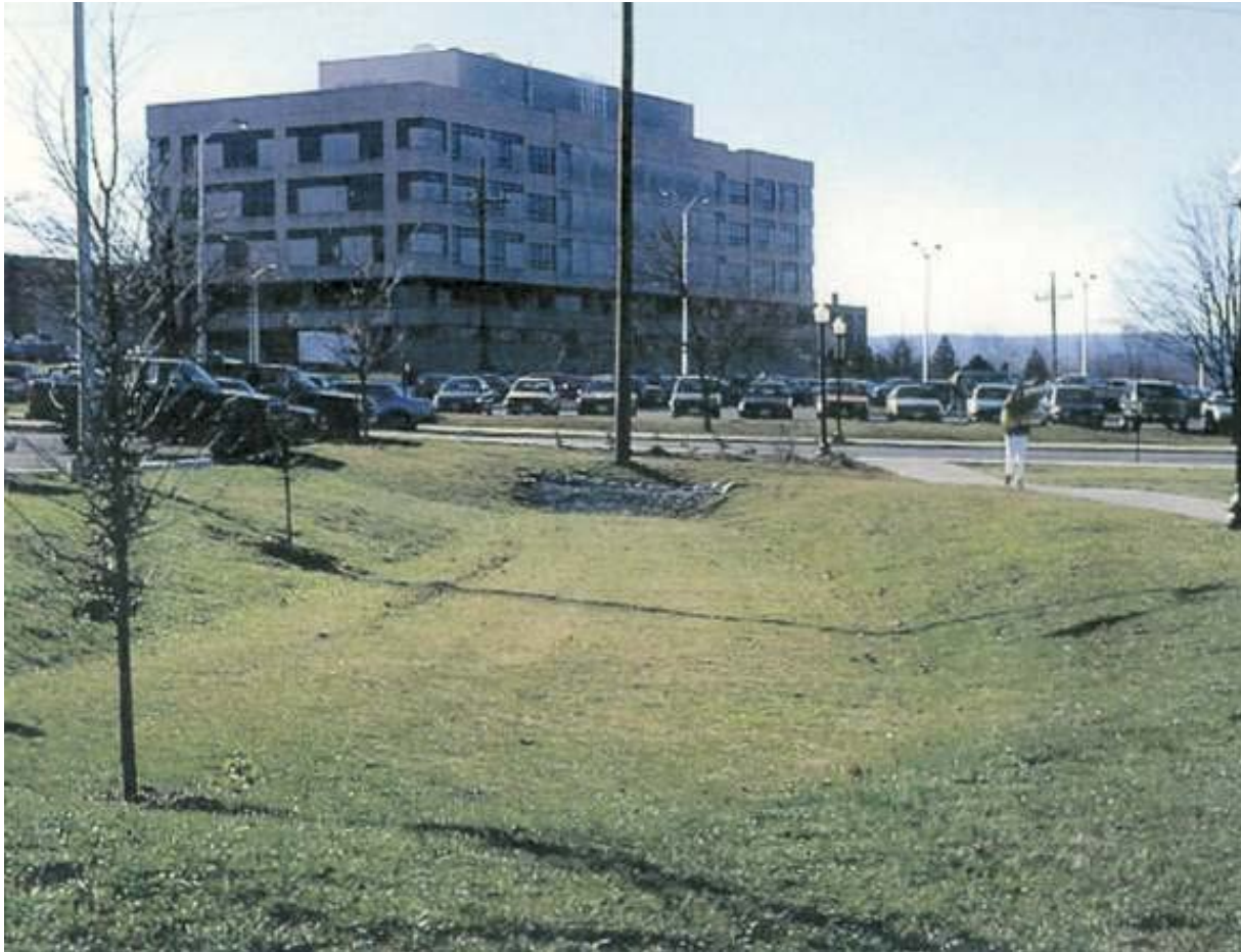
Figure 10.1. Typical Dry Swale in commercial/office setting
