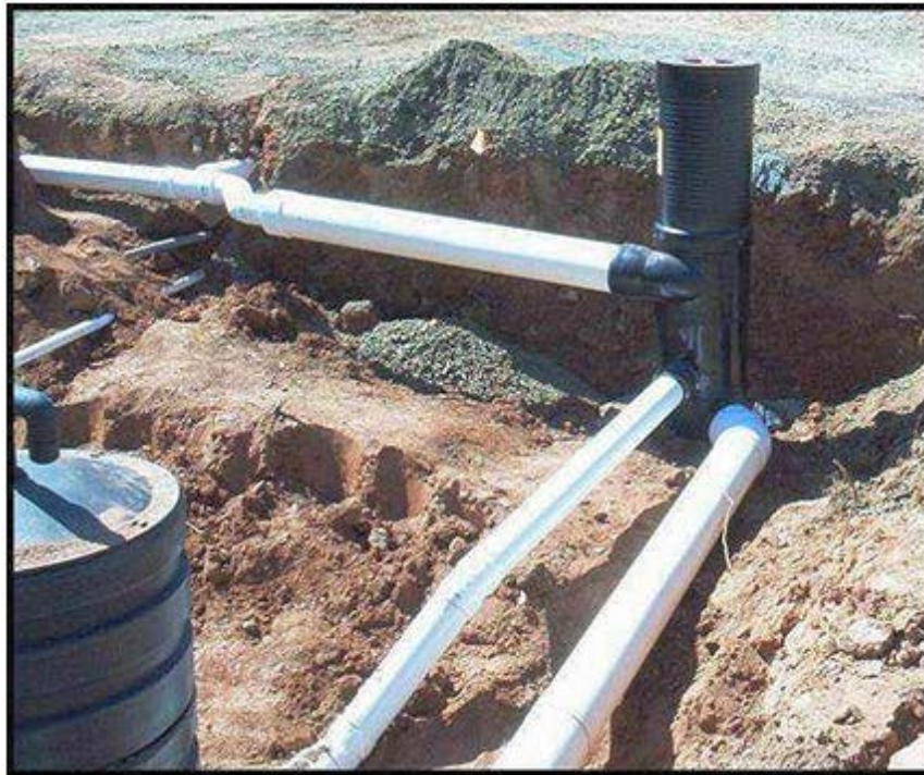
Figure 6.10. Installation of Vortex Filter prior to backfill
